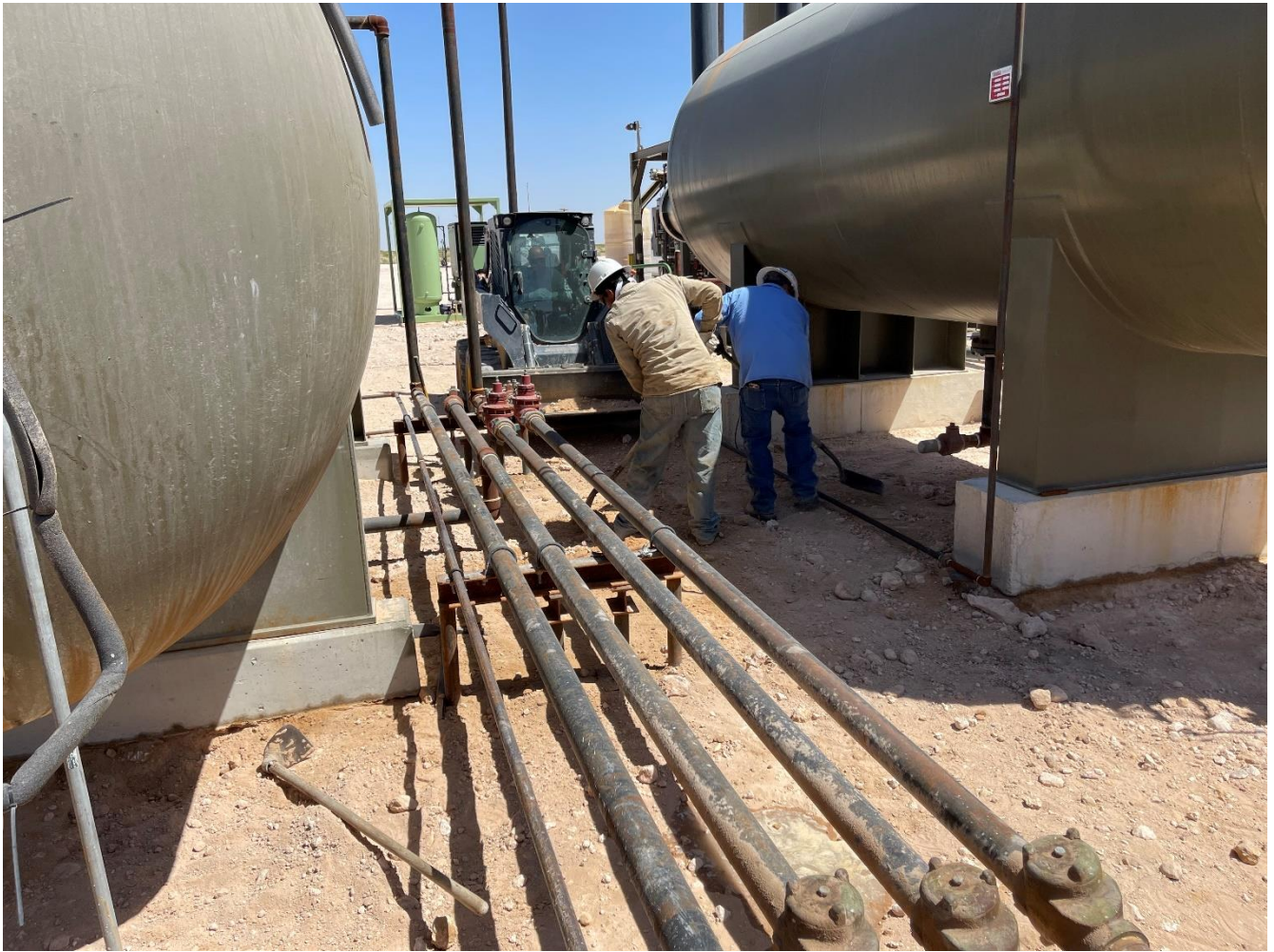
Image 3: Removal of Top Layers of Contaminated Soil Using Skid Steer and Hand Tools in Quadrant 8
