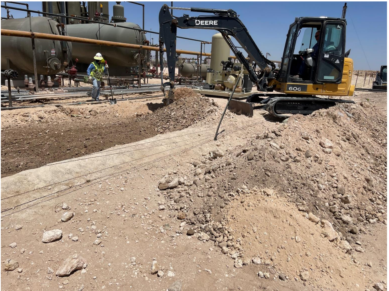
Image 5: Continuing of Removal of Contaminated Soil using Mini Excavator.
