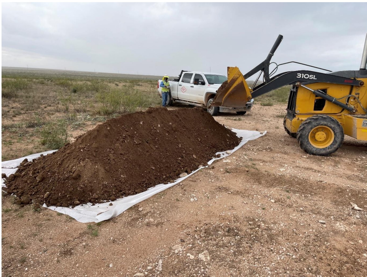
Image 13: Soil removed for Disposal was piled upon plastic sheeting as seen for Quadrants A1 and A10 here
