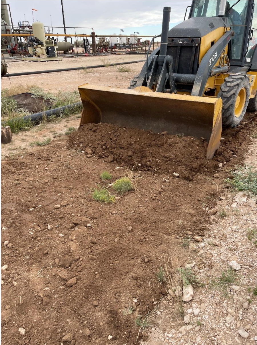
Image 12: Removal of Soil from Surrounding Areas of the Release in Quadrant A1
