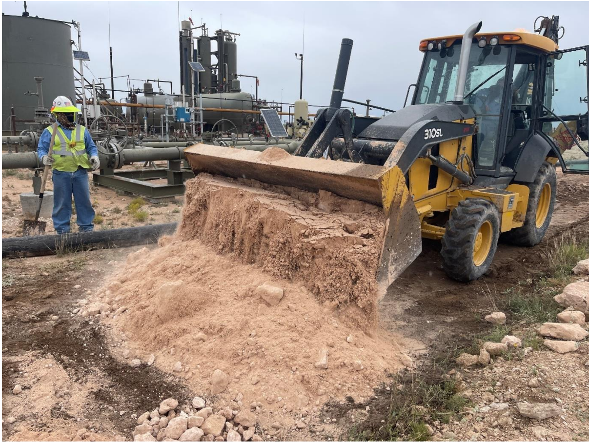
Image 15: Backfill of Surrounding Quadrants with clean soil.
