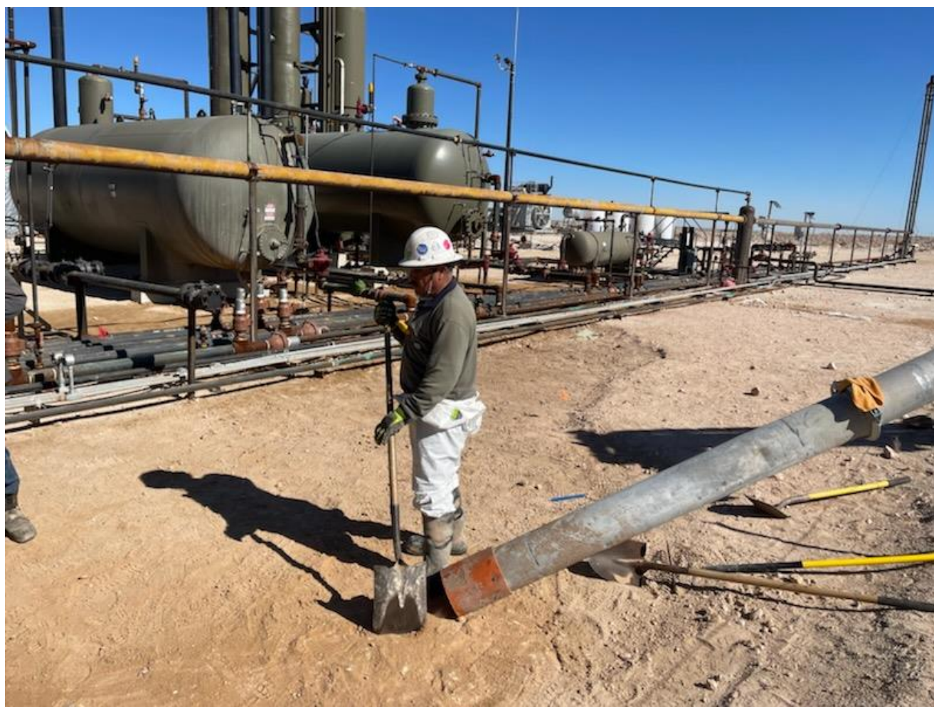
Image 2: Removal of Top Layer of Contaminated Soil Using Hydro-Vac and Hand Tools in hard-to-reach areas such as Quadrant 6 shown here
