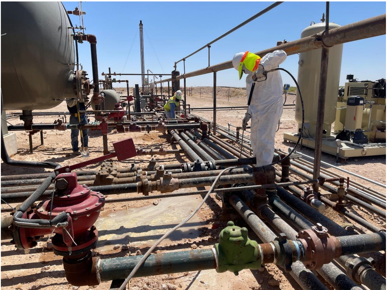
Image 4: Image of Excavation Done on Quadrant 8 Around Pipes using hydro-vac.
