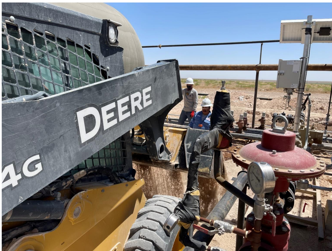
Image 7: Backfilling with Clean Soil Using Skid Steer in Quadrant 8
