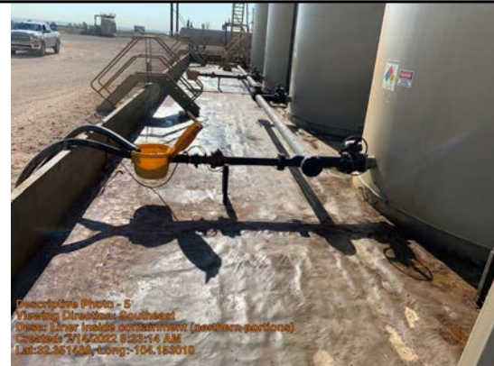
Liner inside containment (northern portions)
