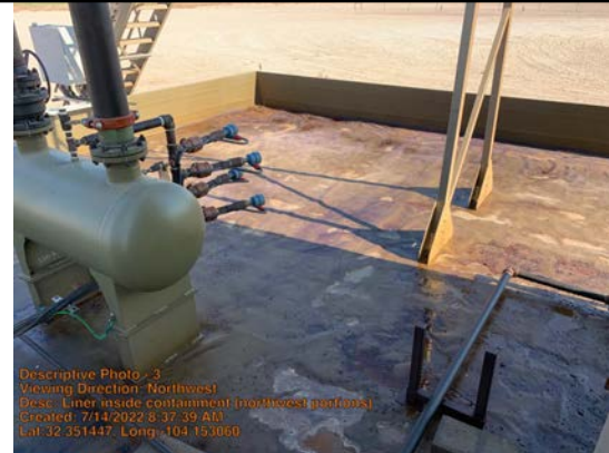
Liner inside containment (northwest portions)
