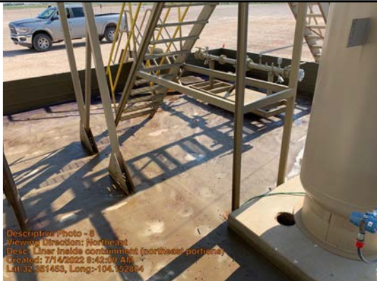
Liner inside containment (northeast portions)
