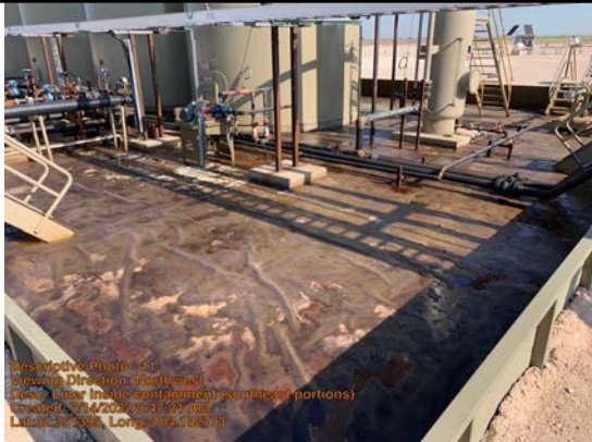
Liner inside containment (southeast portions)
