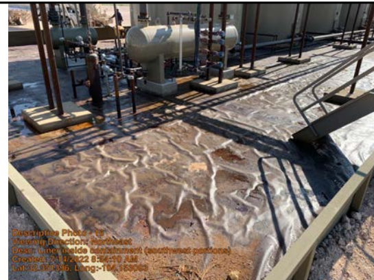
Liner inside containment (southwest portions)
