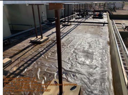
Liner inside containment (southern portions)
