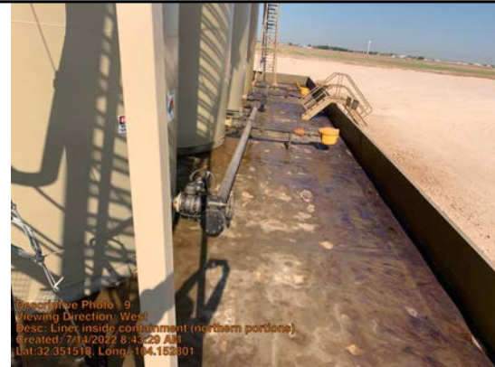
Liner inside containment (northern portions)
