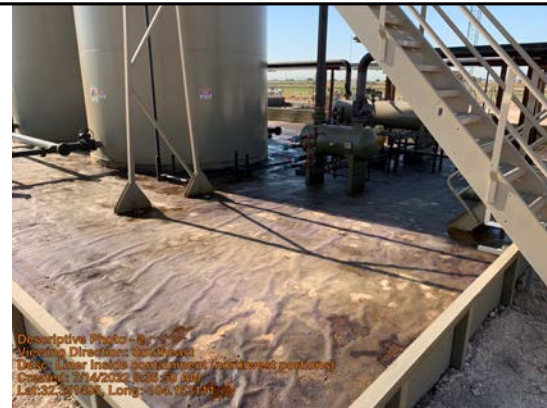
Liner inside containment (northwest portions)
