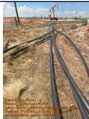
Ground staining beneath poly lines
