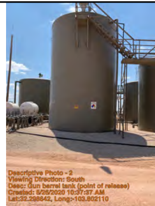
Gun barrel tank (point of release)
