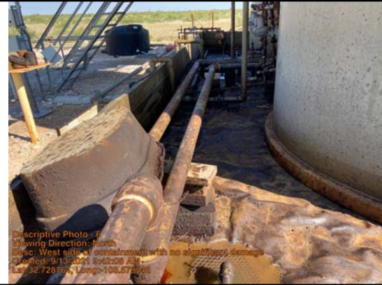
West side of containment with no significant damage
