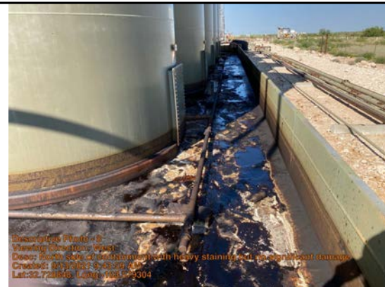
North side of containment with heavy staining but no significant damage
