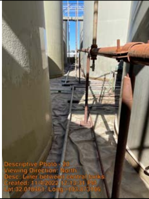
Liner between central tanks.
