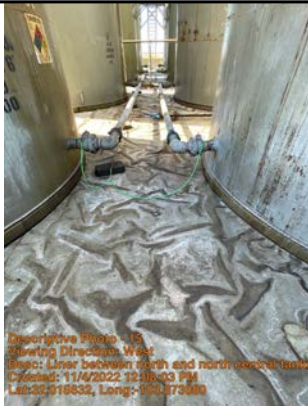
Liner between north and north central tanks
