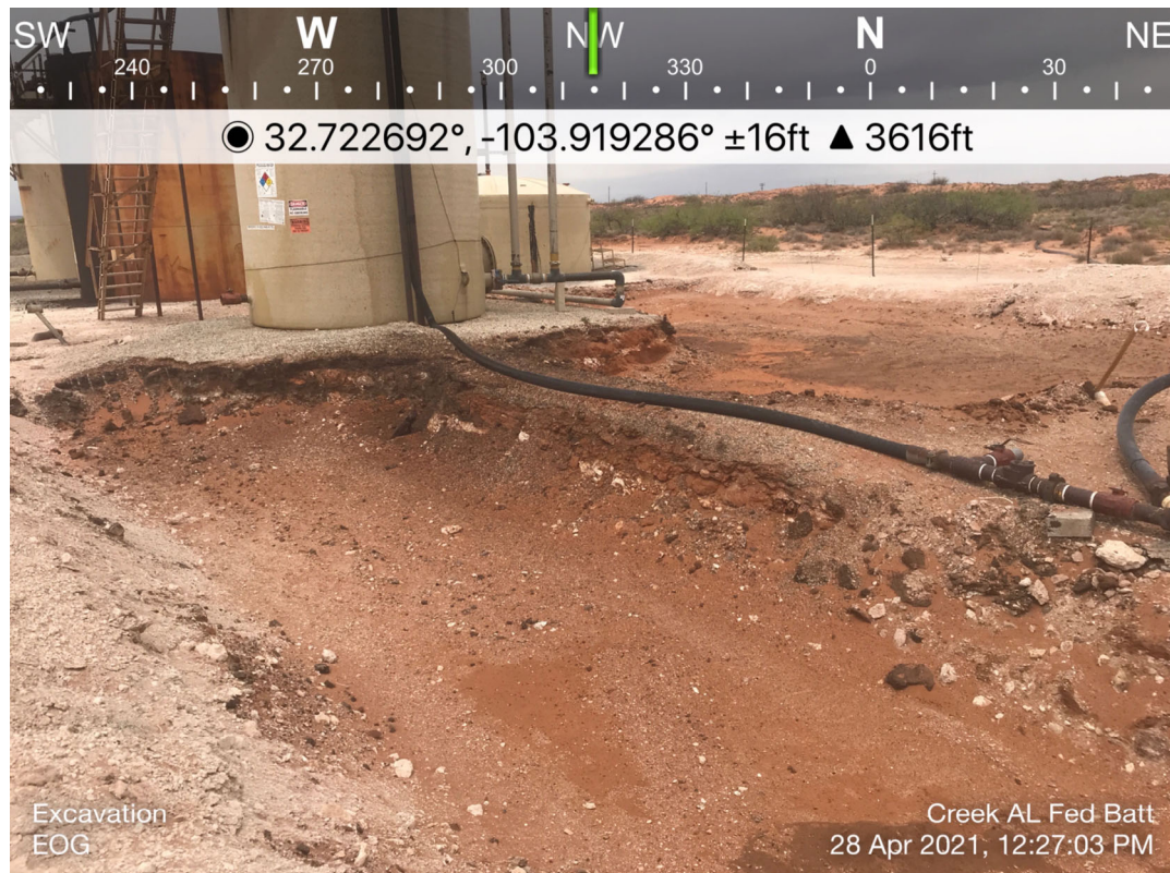
View of Remediation Activities – View Northwest
