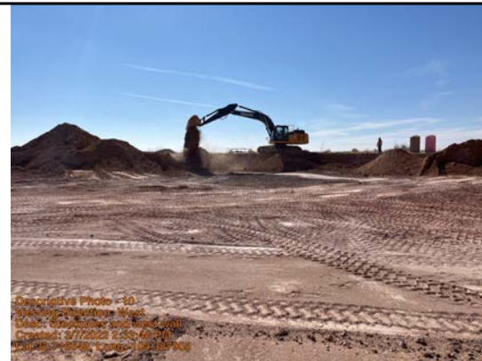
Stockpiles and west wall
