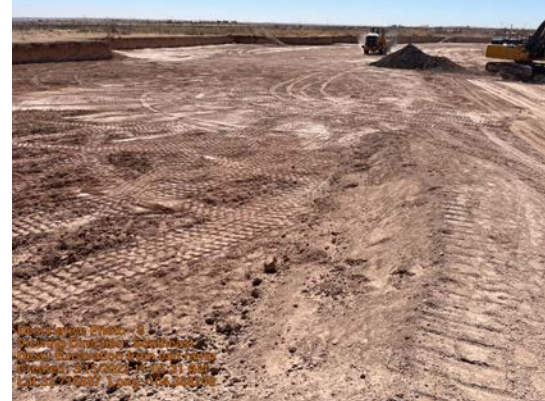
Excavation from exit ramp
