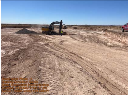
Excavation from exit ramp
