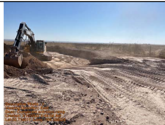
Completed entrance ramp
