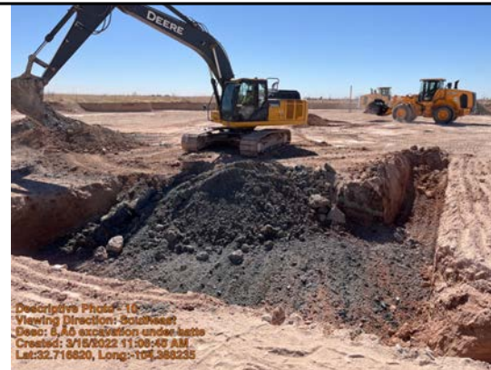
8' excavation under sample points 38 and 41
