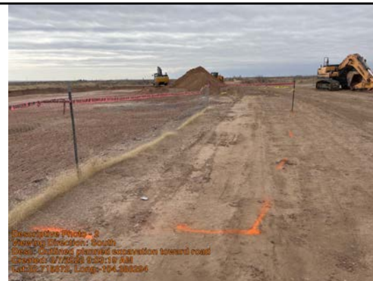
Outlined planned excavation toward road
