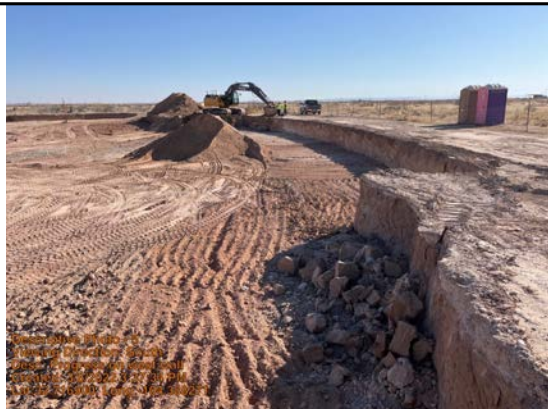
Progress on west wall
