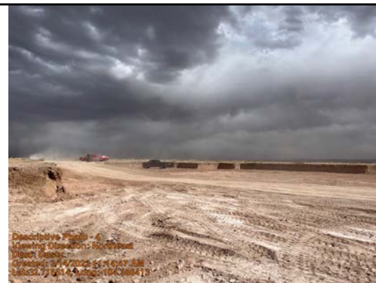
North side of the excavation
