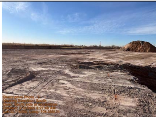
South side of excavation
