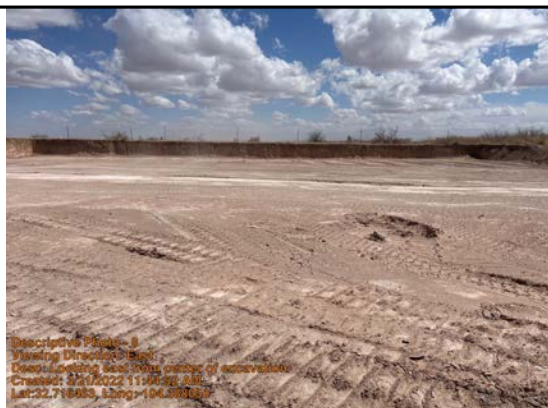
Looking east from center of excavation
