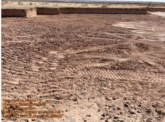
Excavation from exit ramp
