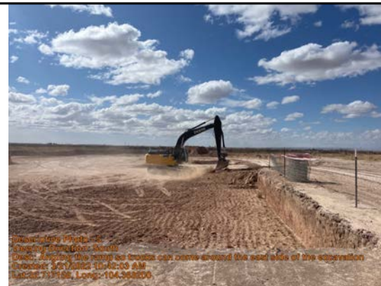
Angling the ramp so trucks can come around the east side of the excavation
