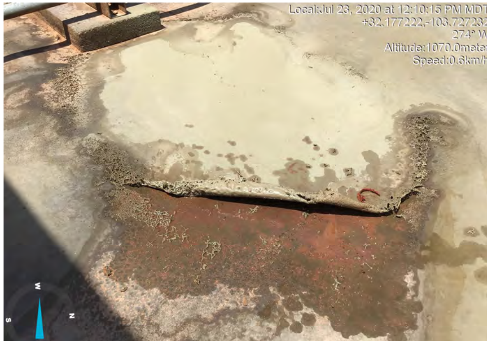
West side inside (pump#1), patch unglued
