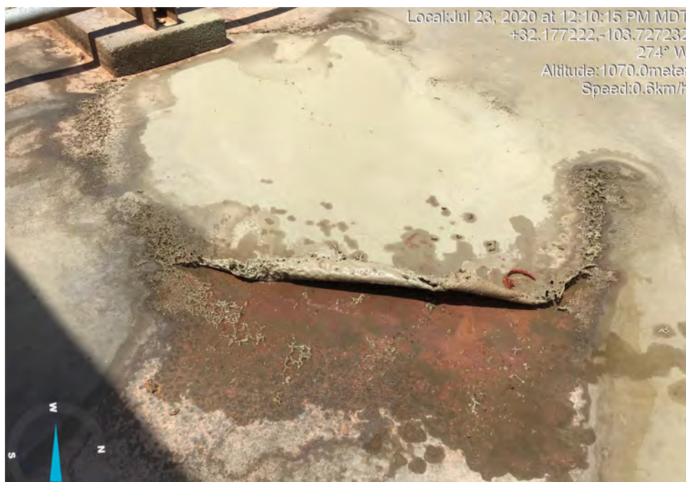
West side inside (pump#1), patch unglued
