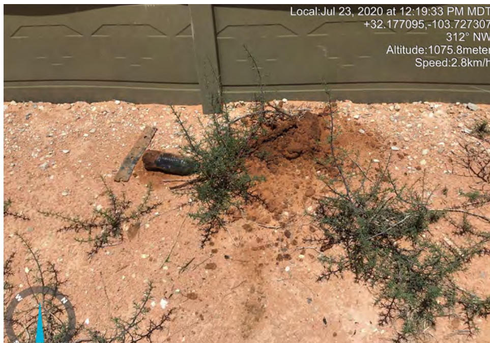
East side, outside of liner, oil stain (not liner leak), oil dump
