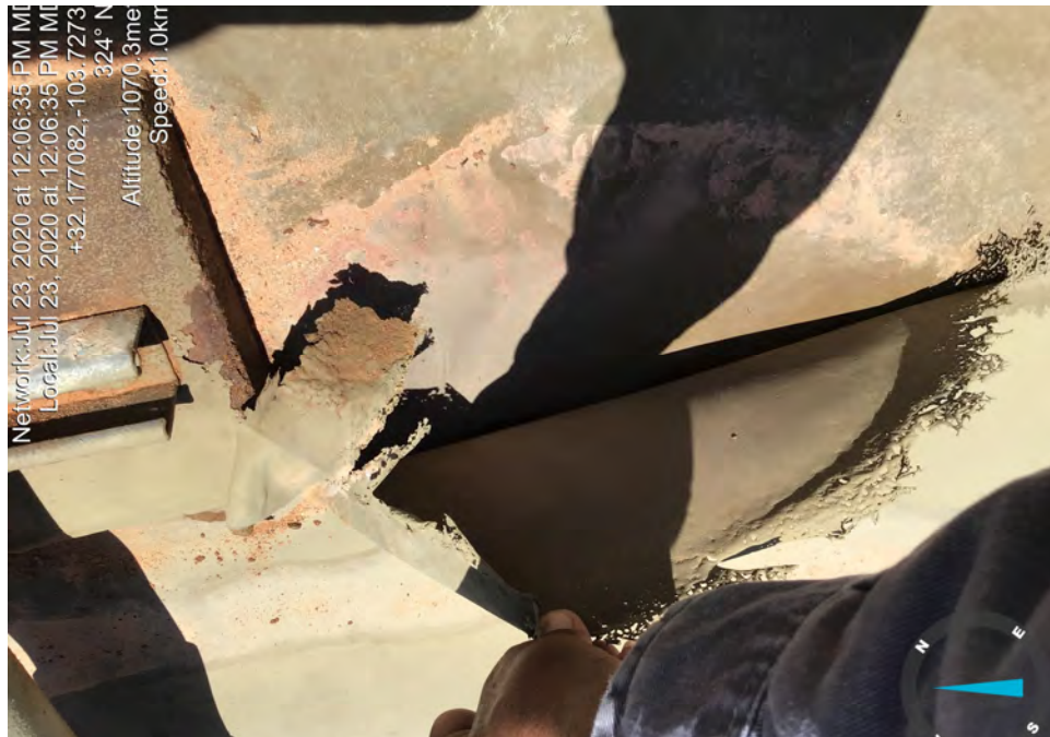
East side, inside pump#3, liner patch unglued
