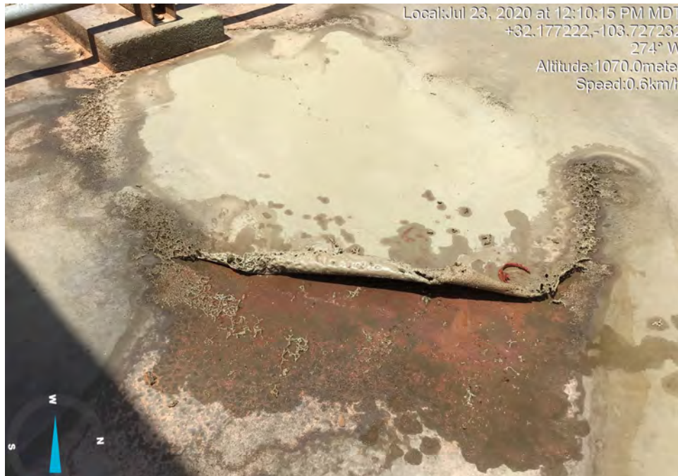
West side inside (pump#1), patch unglued
