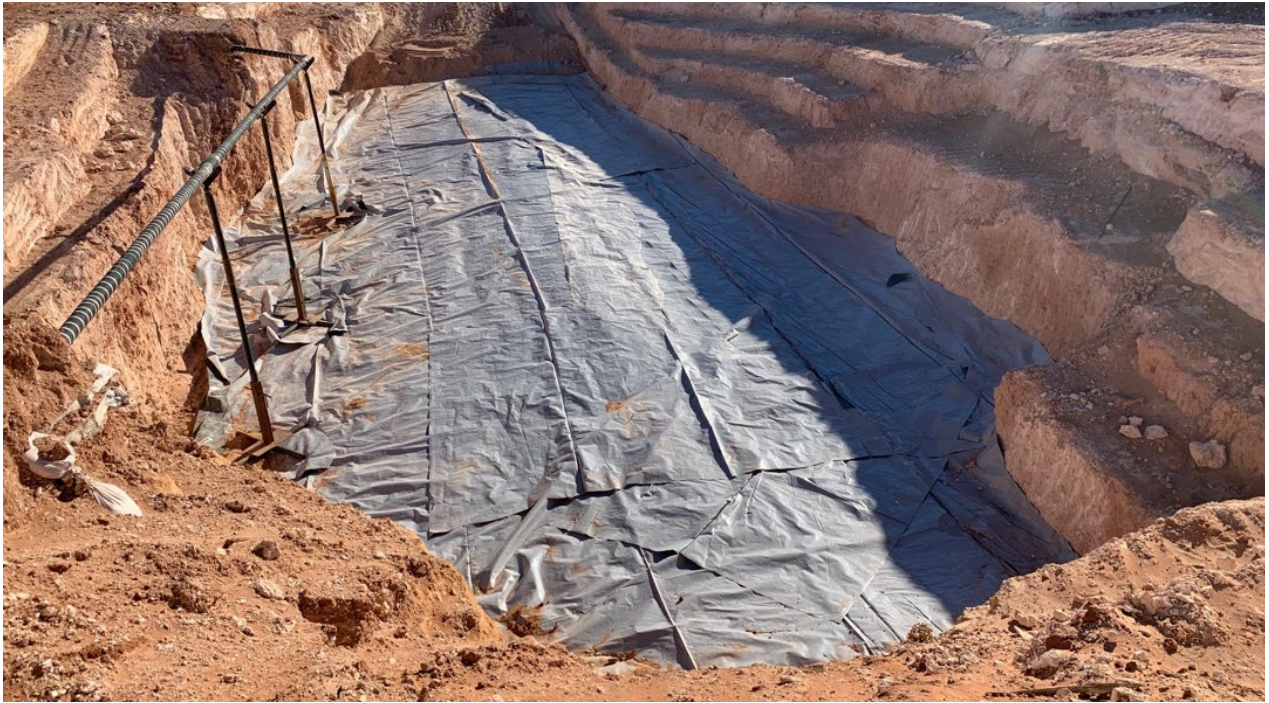
Photo 7 View to the east following liner installation activities.
