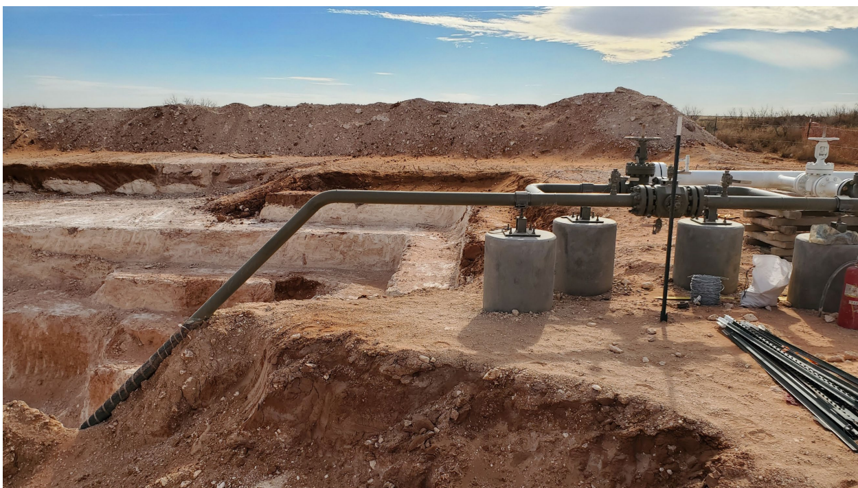
Photo 4 Plains pipeline and riser on the west side of the excavation.
