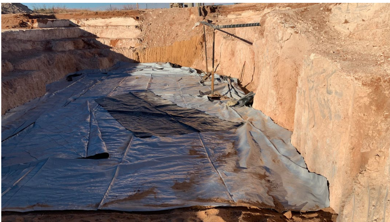
Photo 6 View to the west at the excavation with the liner being installed.
