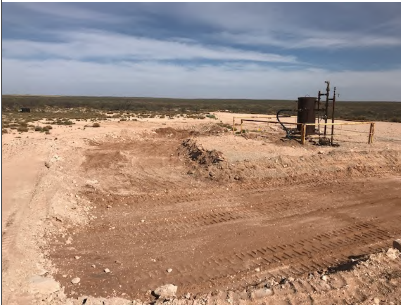
View of the northern excavation area.
