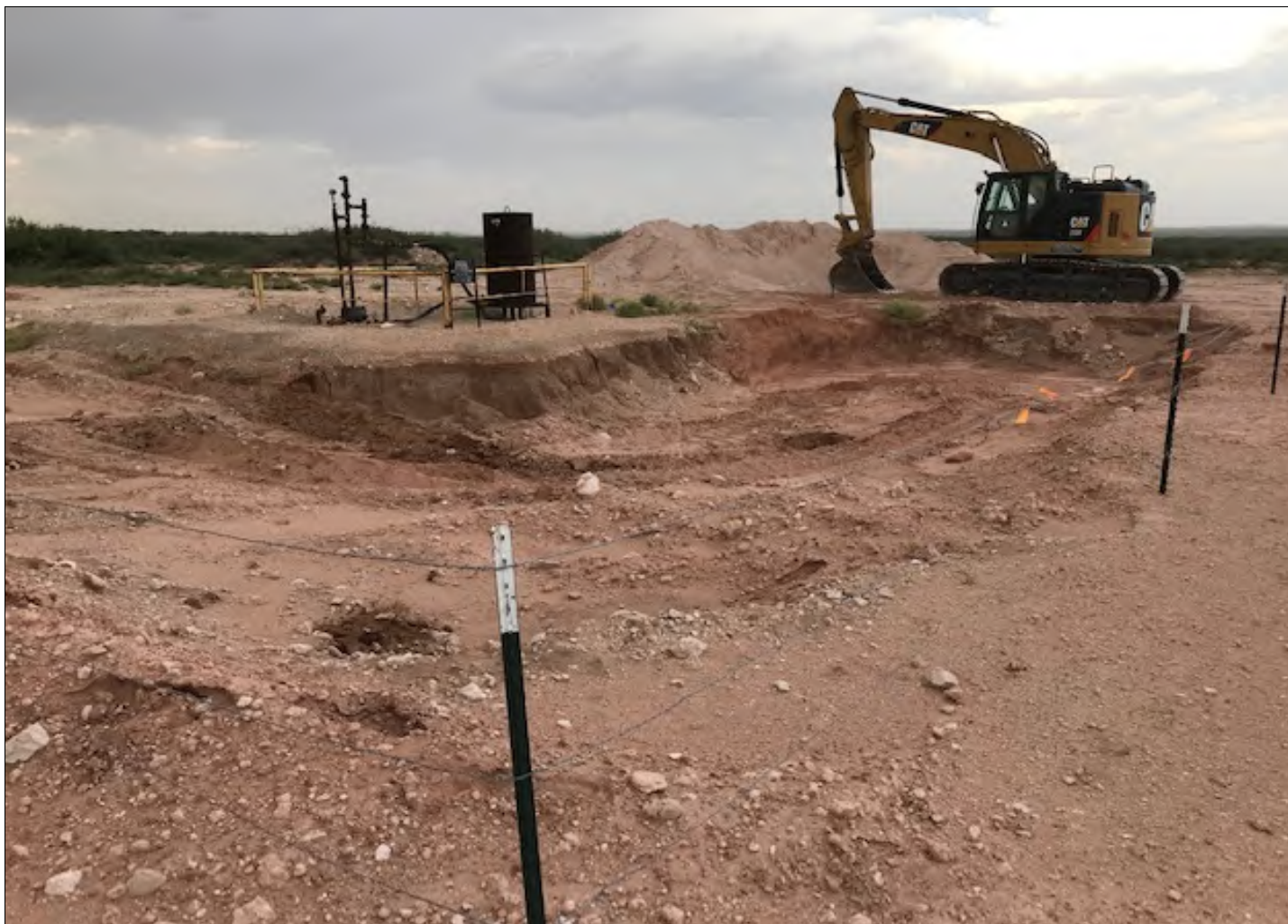
View of the southern excavation area.
