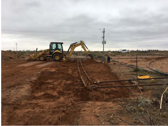
Continue backfilling.
