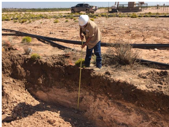
Excavating to a depth of 4' bgs.
