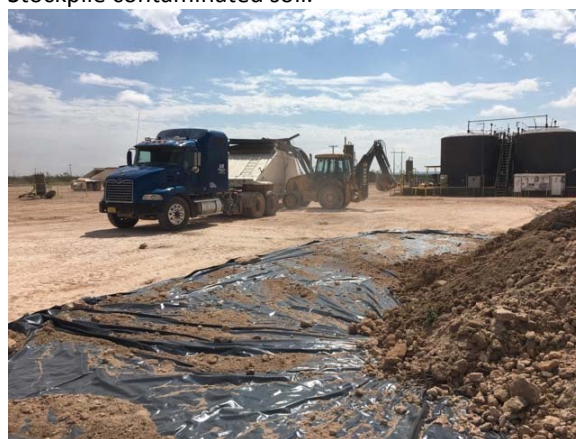
Stockpile contaminated material on liner.
