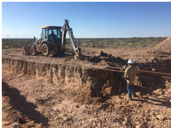
Install T-Post to hold lines.
