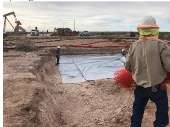
Began installing and backfilling 20 ml liner in sections.
