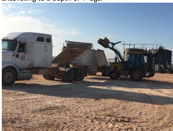
Load and export contaminated soil.
