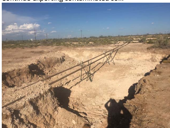
Continue installing T Post and excavating under lines.
