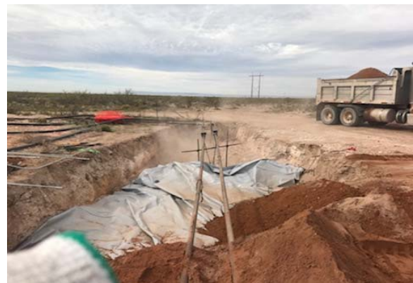
Backfilling excavated area.
