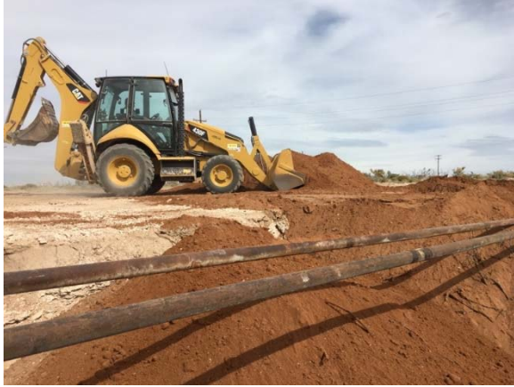
Continue backfilling.
