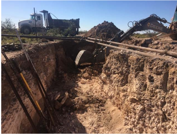
Excavating under lines.
