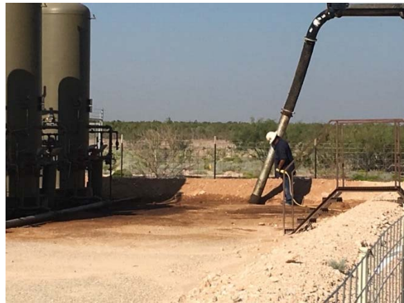
Utilizing hydro vac to excavate release area
