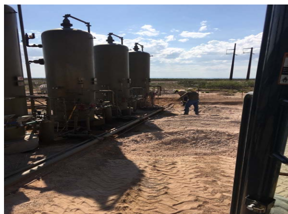
Begin backfilling excavation area
