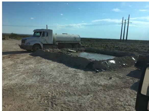
Lined spoil area containment
