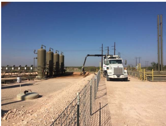
Utilizing hydro vac to excavate release area
