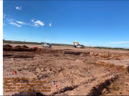
Final excavation pad
