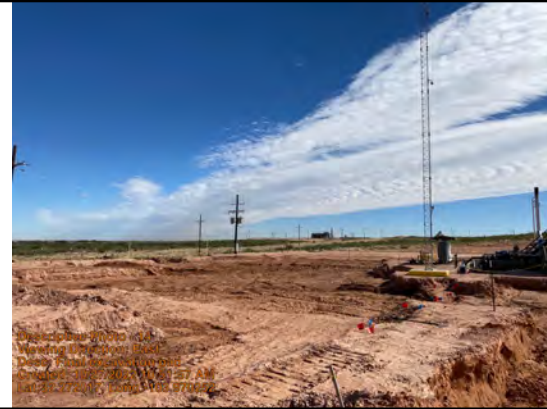
Final excavation pad
