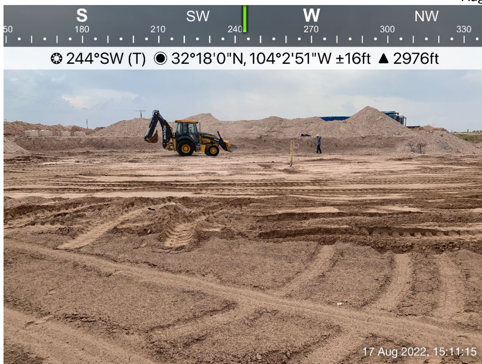
Backfilled excavation viewing southwest, August 17, 2022
