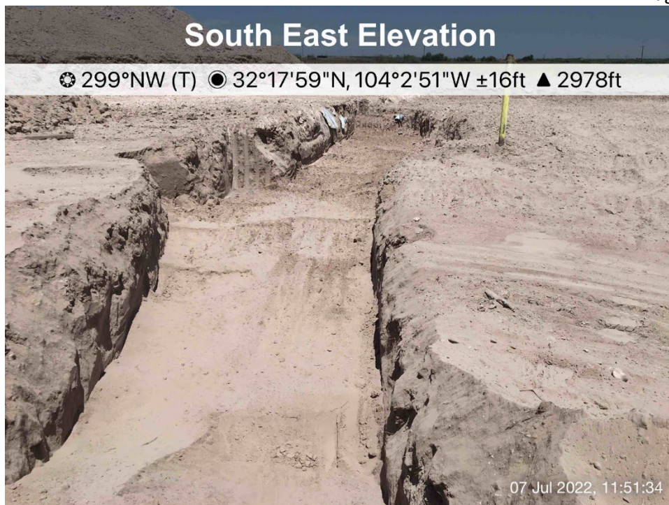
Excavated area viewing northwest, July 7, 2022
