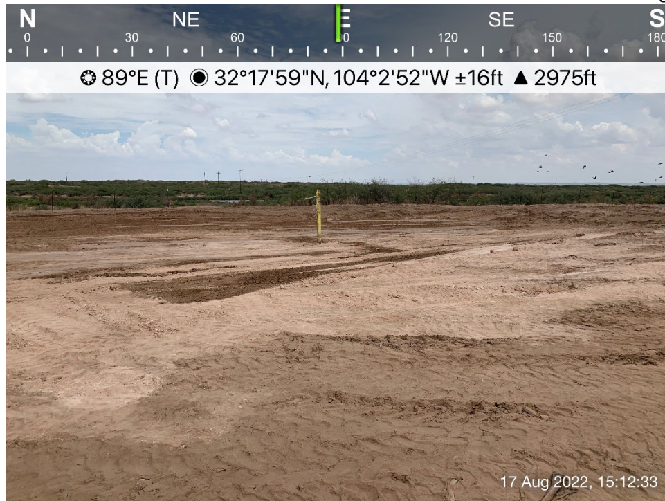
Backfilled excavation viewing east, August 17, 2022
