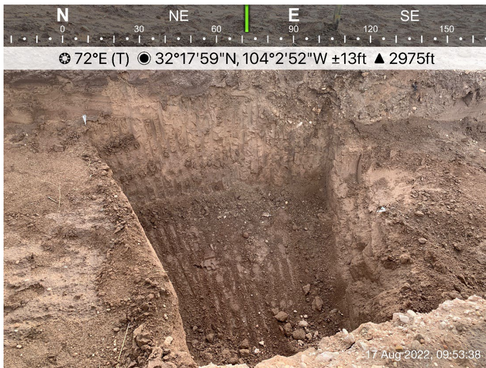
Additional excavated soil encompassing C-23, August 17, 2022
