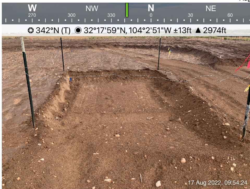
Additional excavated soil encompassing C-13, August 17, 2022
