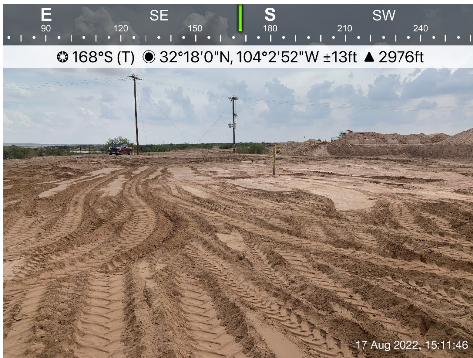
Backfilled excavation viewing south, August 17, 2022
