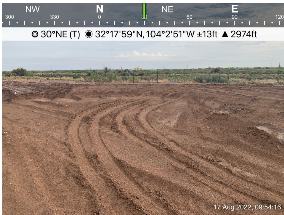
Additional excavated soil encompassing C-27, August 17, 2022
