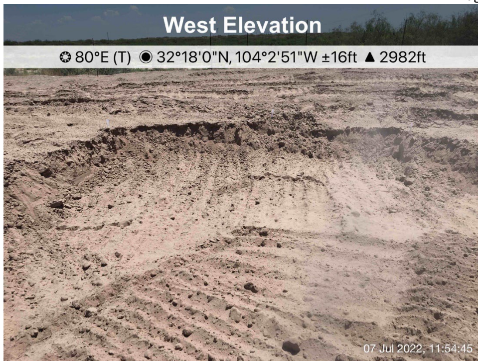
Excavated area viewing east, July 7, 2022
