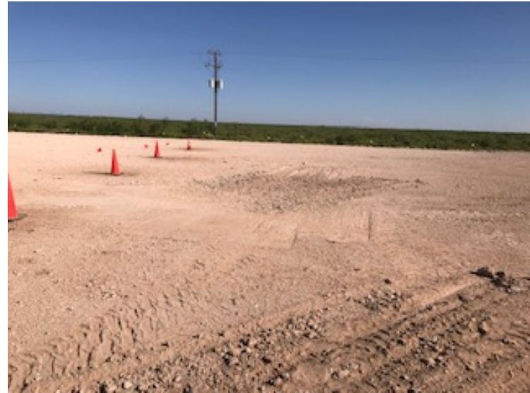
Photograph 6: View of well pad facing south.
