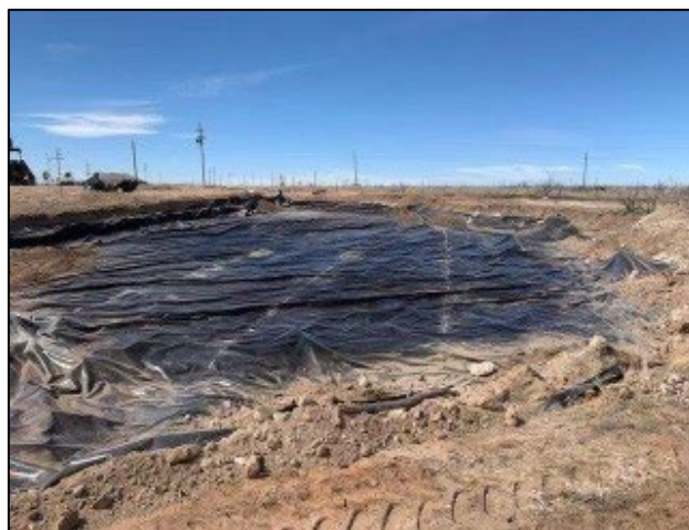
Photograph 2 Date: 03/01/2023 Description: Liner Installation.
