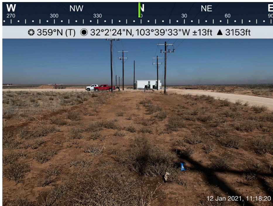
Impacted area (nRM2032861231) viewing North, January 12, 2021
