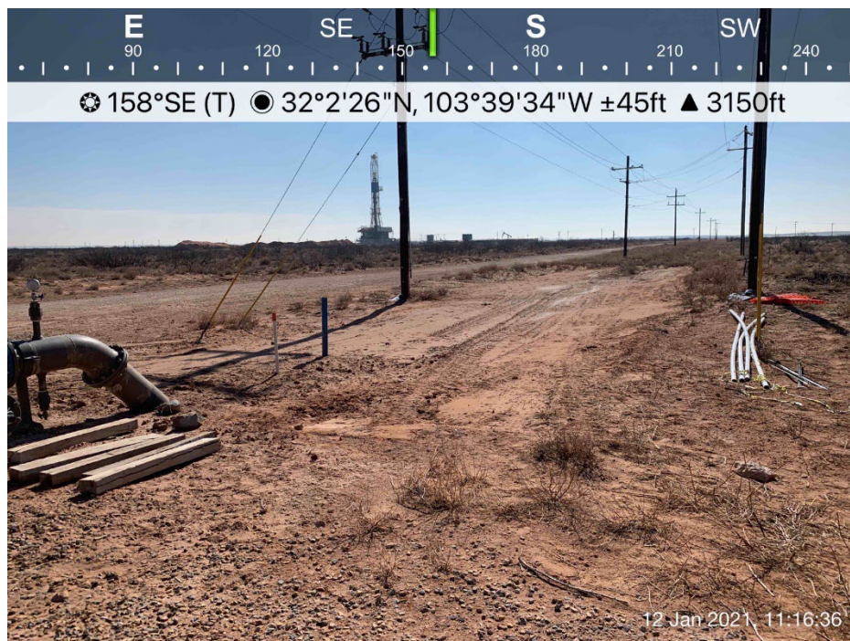
Impacted area (nRM2032861231) viewing Southeast, January 12, 2021
