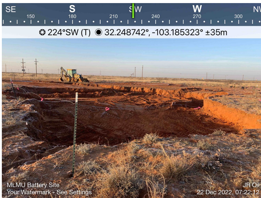
View of Remediation Activities – View Southwest
