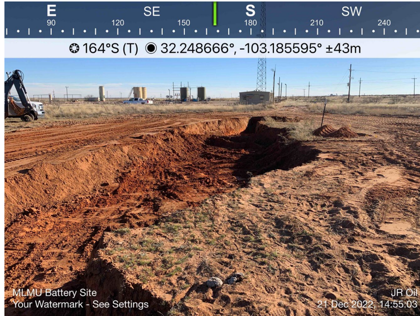
View of Remediation Activities – View South
