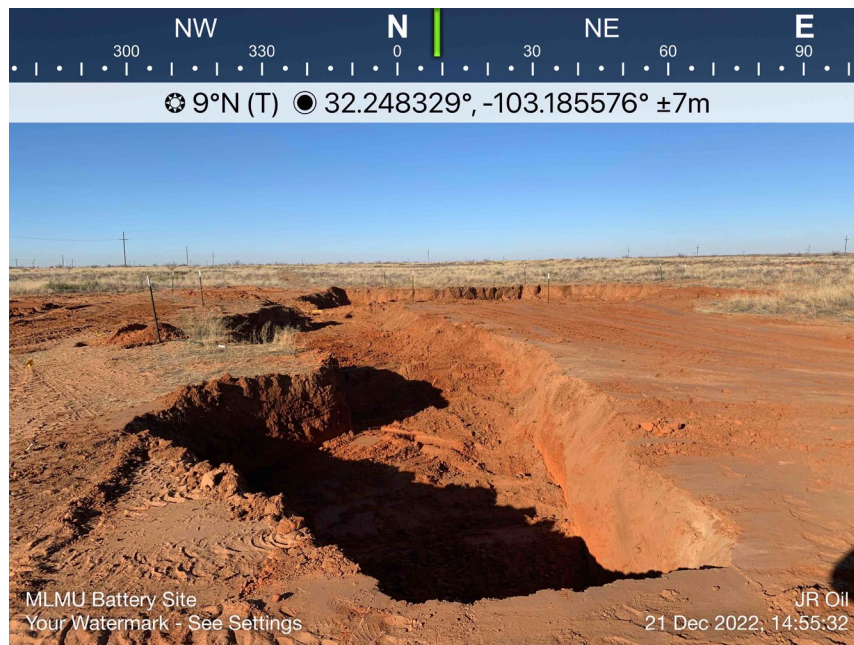
View of Remediation Activities – View North
