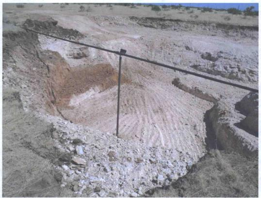
Photograph No. 6 – Looking northerly at excavation, steel pipeline with pipe support and ingress/egress ramp
