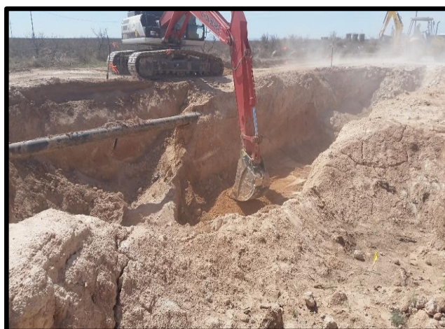
View of hydrocarbon stain removal in the vicinity of the former 30137 #3 excavation, facing southwest.
