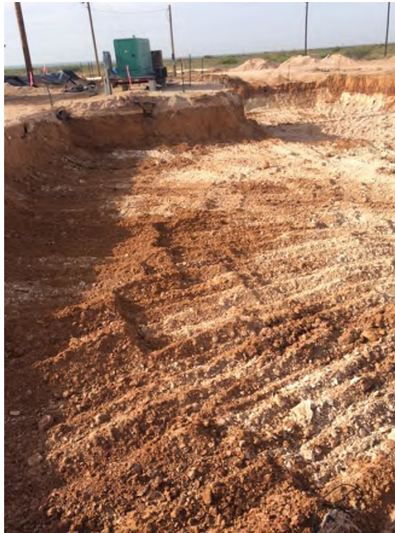
View South – Excavated area of the former facility
