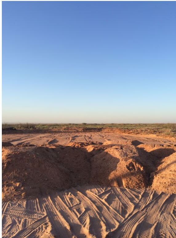
View West- Backfilled area of the West Spill
