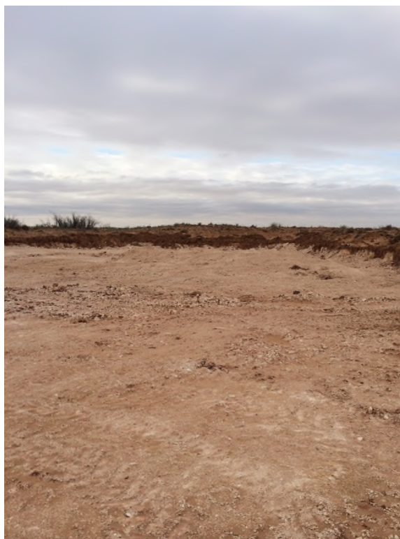
View South – Excavated area of the South Spill
