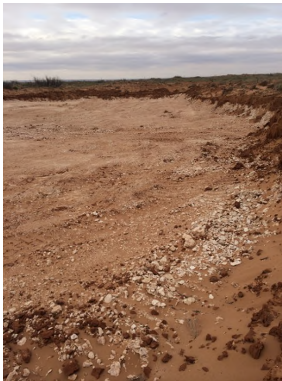
View West – Excavated area of the West Spill
