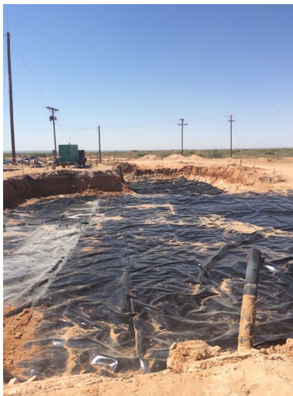
View South – Lined area of the former facility
