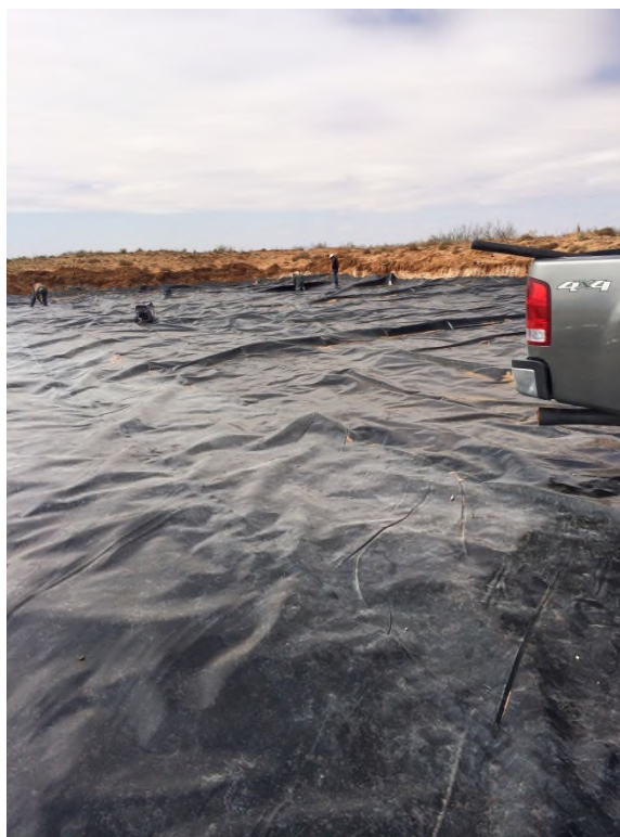
View West – Lined area of the West Spill
