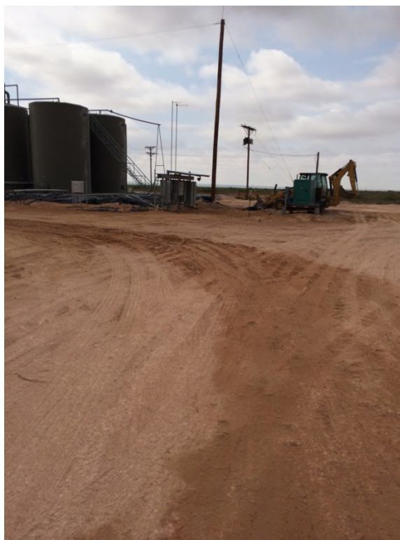
View South – Backfilled area of the former facility
