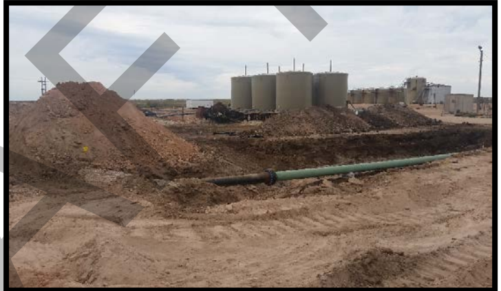
View of stockpiled soils generated during over-excavation activities, facing northeast.
