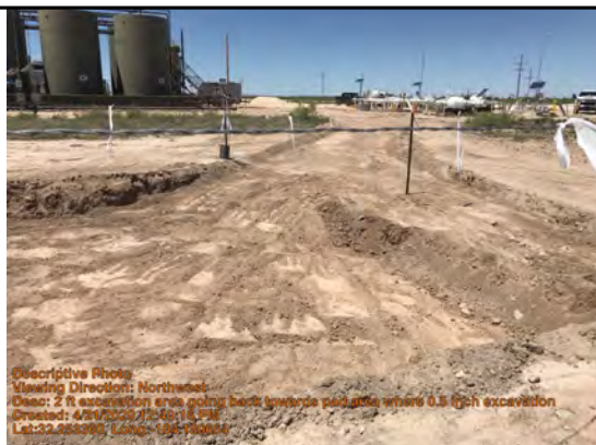
2 ft excavation area going back towards pad area where 0.5 inch excavation occurred
