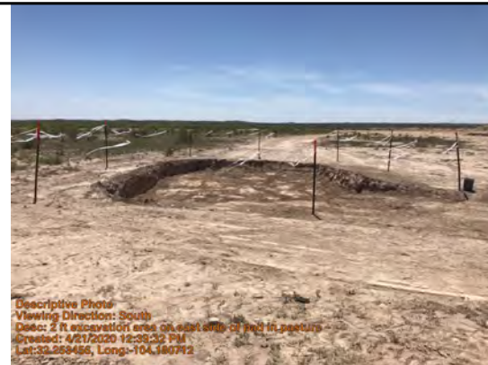
2 ft excavation area on east side of pad in pasture
