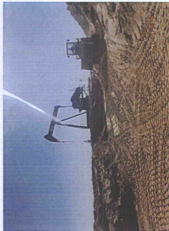
Backfilling base of excavation with caliche, facing south
