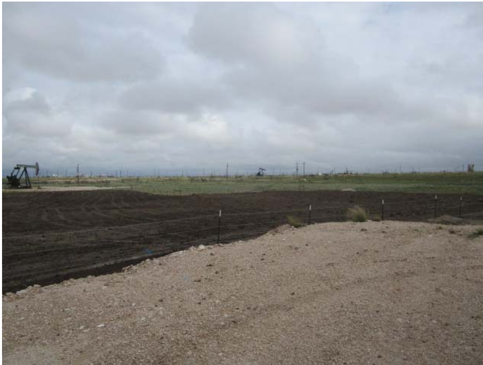
Photo 11 - A foot of topsoil placed and reclaimed area fenced off for seeding
