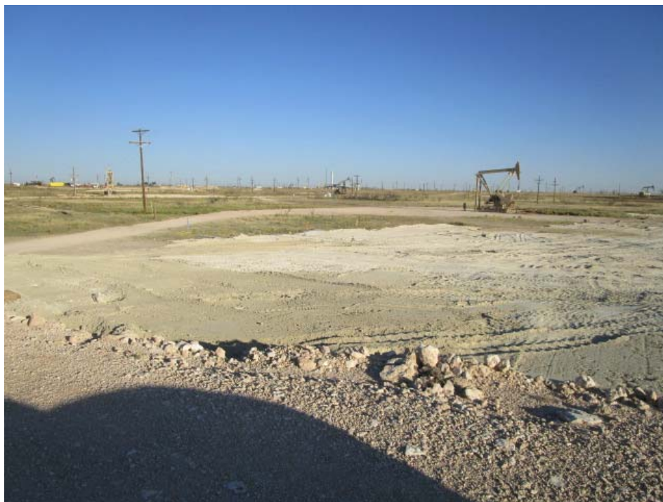
Photo 9 - Approximately one foot of caliche placement complete
