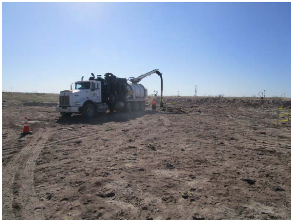
Photo 2 - Locating underground pipelines via hydrovac
