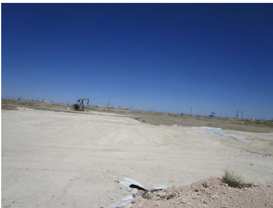
Photo 8 - Caliche placed on top of the liner to secure in place
