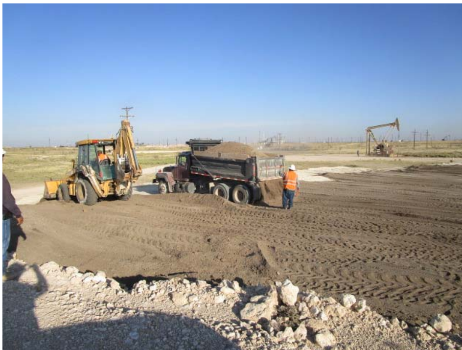
Photo 10 - Placement of topsoil on caliche
