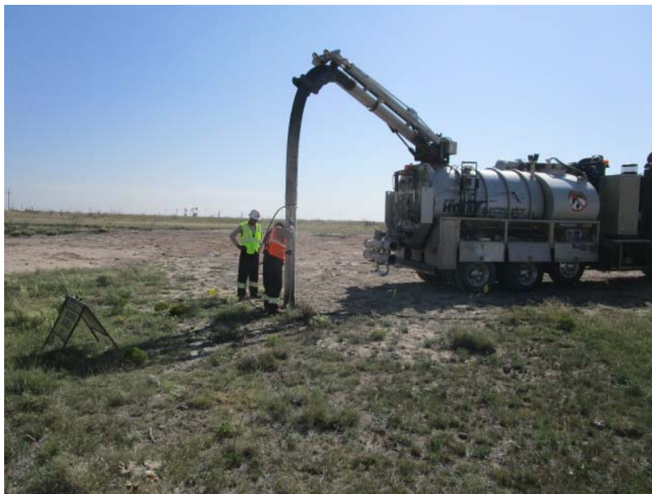
Photo 1 - Locating underground pipelines via hydrovac
