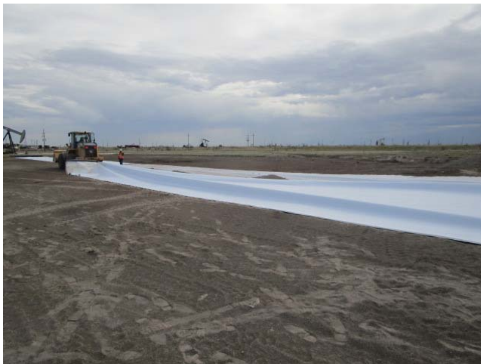
Photo 5 - Liner being placed
