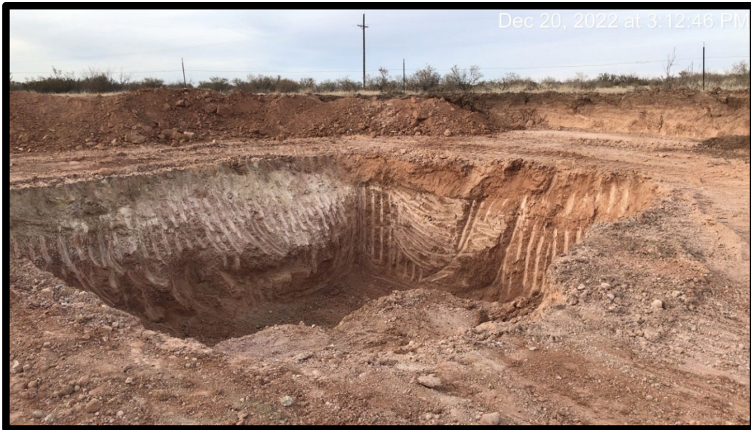
PHOTOGRAPH NO. 5 – A view of the excavation area completed to a maximum depth of approximately 15 feet bgs. The view is towards the northwest.
