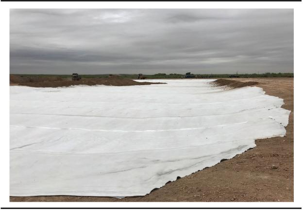
Figure 9 - View of installation of the bentoliner, facing north.
