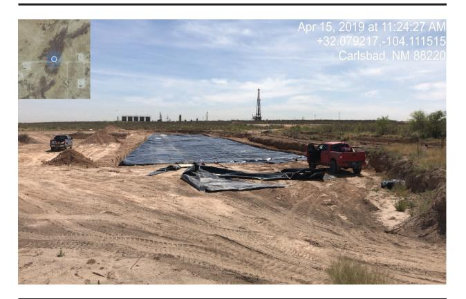
Figure 3 - View of installed polyuruthane liner, facing east.
