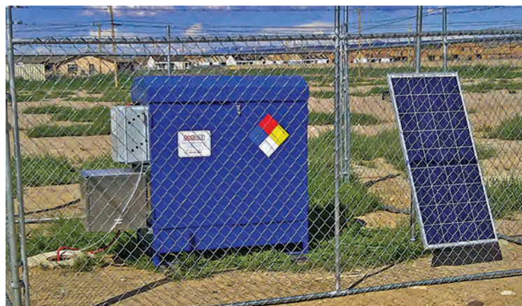
Solar Sipper installation mounted on hazmat enclosure
