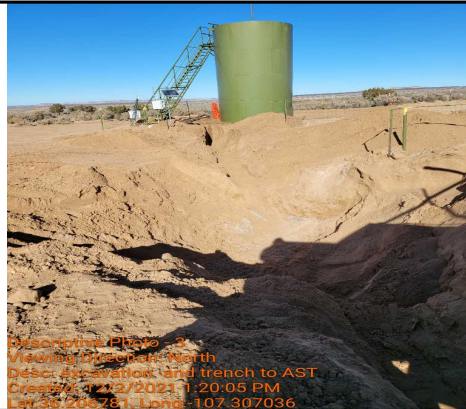
excavation and trench to AST
