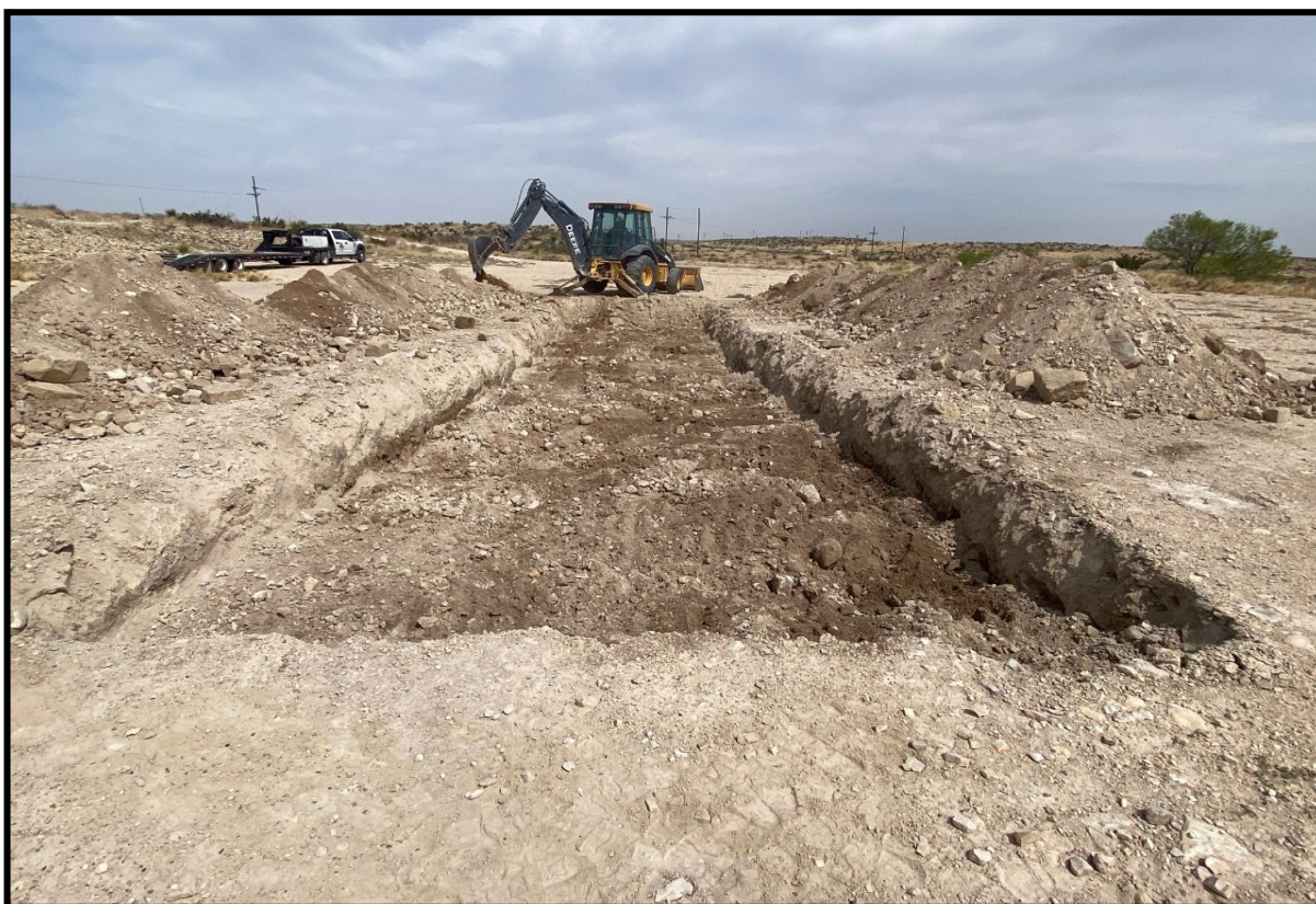
View of the final excavation of impacted soils from the release area, facing northwest.
