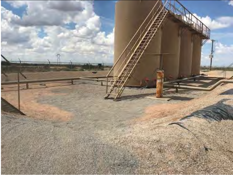
Photo 11: View southwest of the backfill of the lined secondary containment area. Clean pea gravel was placed over the repaired liner.
