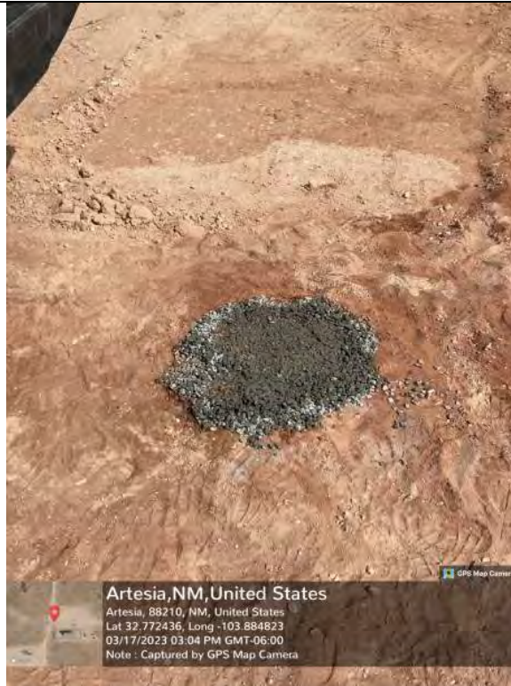
Photo 15: View of TMW-1 plugged after gauging (no water).
