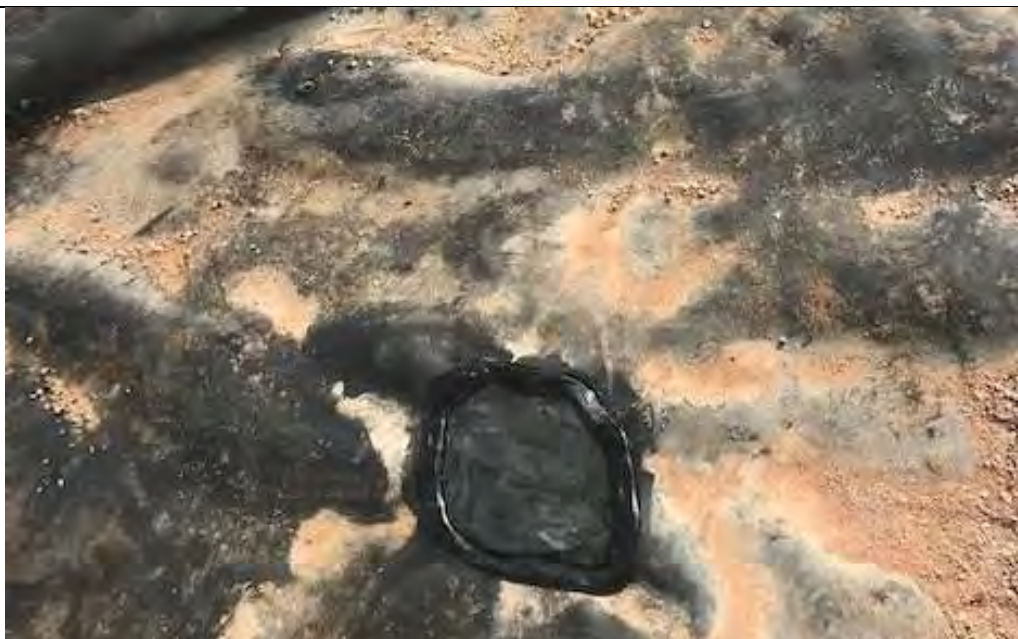
Photo 10: View of the repaired liner in the S-2 area. The secondary containment liner has been repaired, inspected, and determined to be in good condition. The repaired liner will prevent vertical migration of COCs left in situ.
