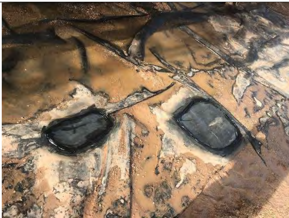
Photo 9: View of the repaired liner in the S-4 and S-5 area. The secondary containment liner has been repaired, inspected, and determined to be in good condition. The repaired liner will prevent vertical migration of contaminants of concern (COCs) left in situ.
