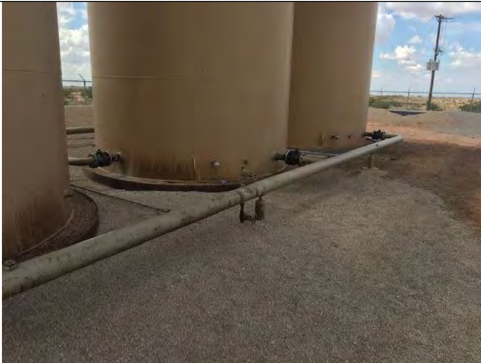
Photo 12: View southwest of the backfill of the lined secondary containment area. Clean pea gravel was placed over the repaired liner.
