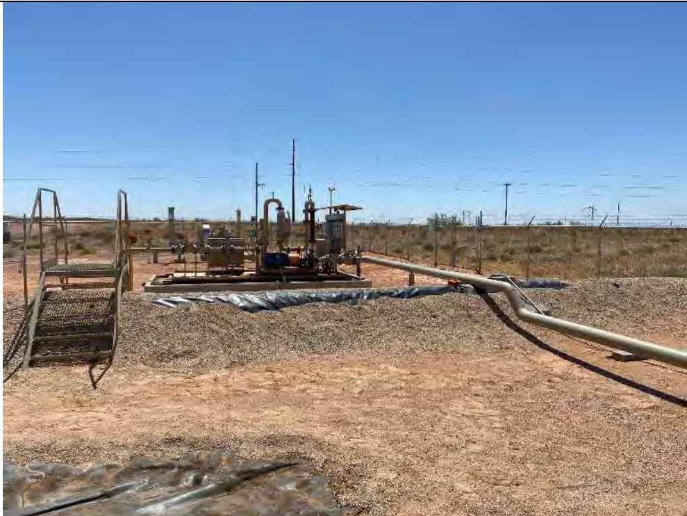
Photo 4: View east of the pump and associated pad, with aboveground steel piping extending into the lined secondary containment area.
