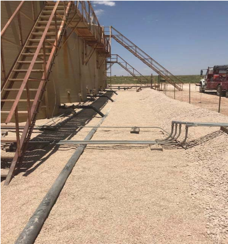
View North – Remediation activities (backfill) completed inside secondary containment.
