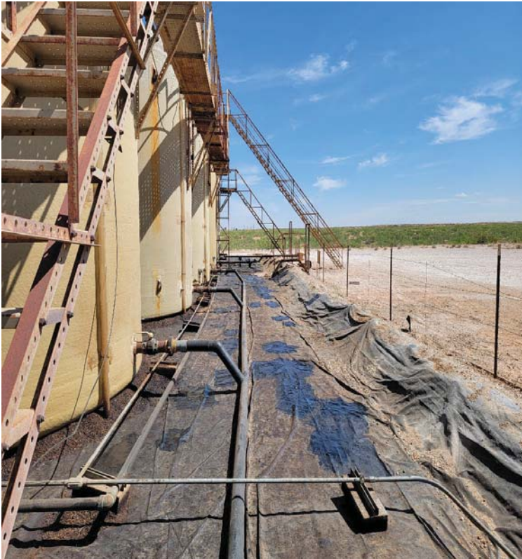
View North – Remediation activities (pressure washing and excavation) completed inside secondary containment.
