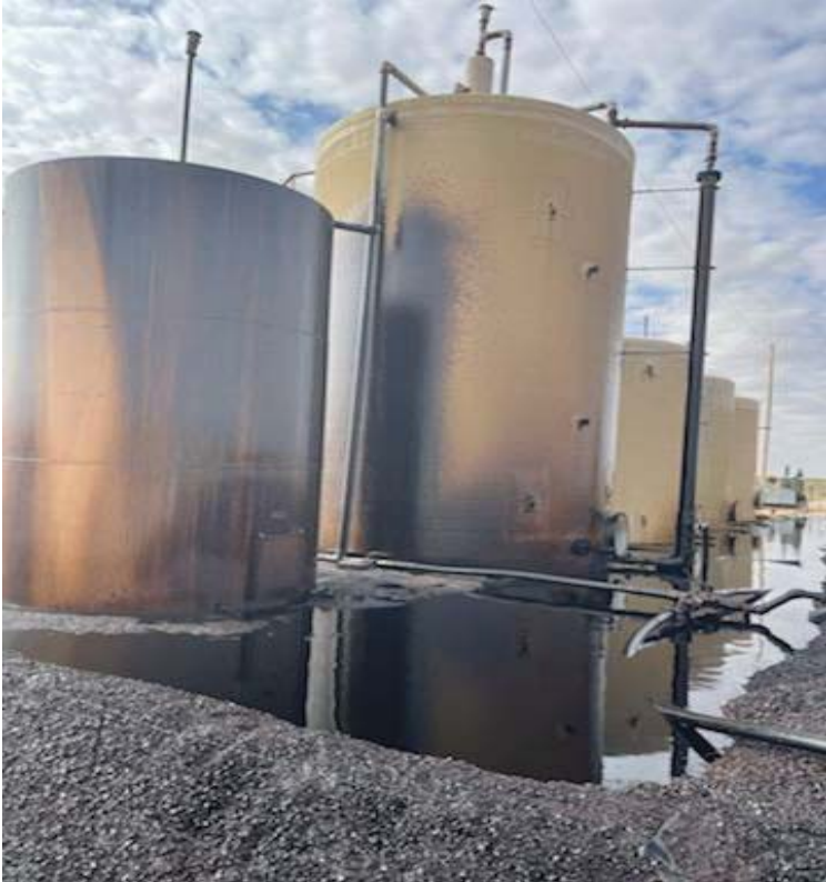
View South – Origin of spill. Cause of the release is due to a closed valve on the back of the gun barrel (vandalism) causing tanks to overflow.
