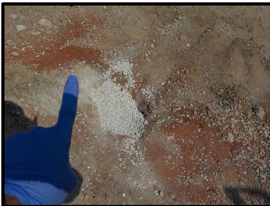
PHOTOGRAPH NO. 2 – A typical view of the soil boring plugging and abandonment activities following installation and sampling.
