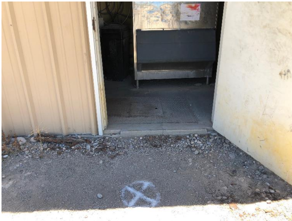
Photo 9 - Looking south at location of DP-15 marked in white near north end of Building 6
