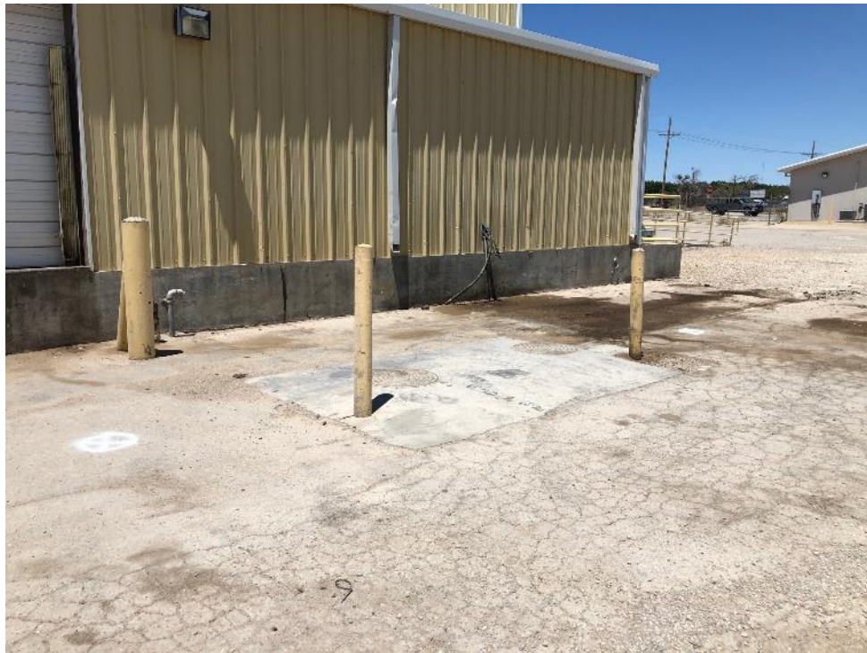
Photo 6 - Looking northwest at east side of building 3 at DP-10 and DP-11 marked I white. Final location of both borings was shifted east to avoid underground piping
