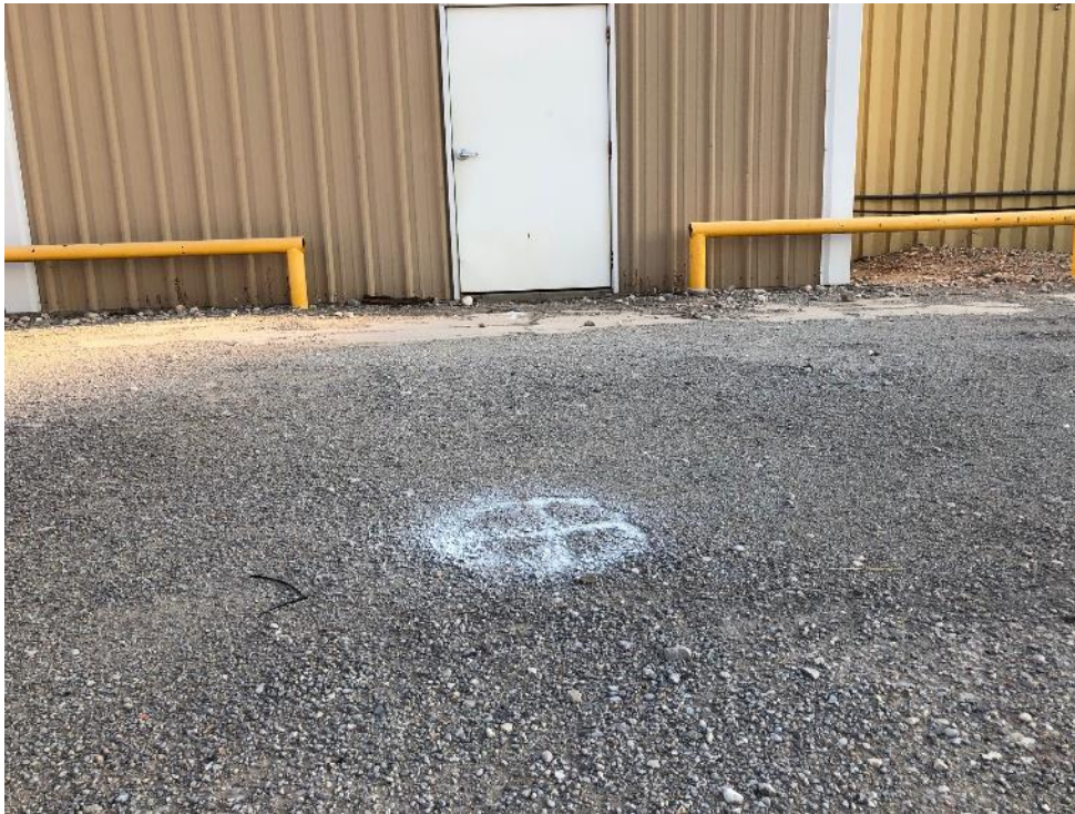
Photo 11 - Looking south at location of DP-18R marked in white north of Building 6
