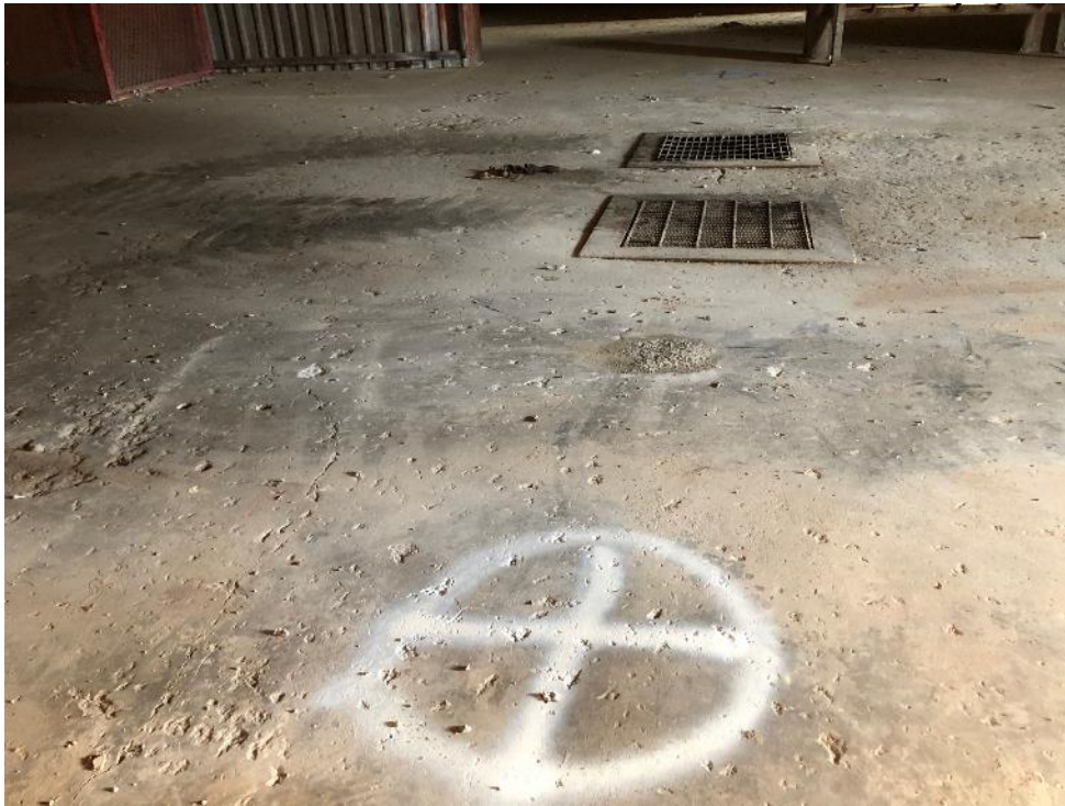
Photo 13 - Looking south at location of DP-20R marked in white inside of Building 6
