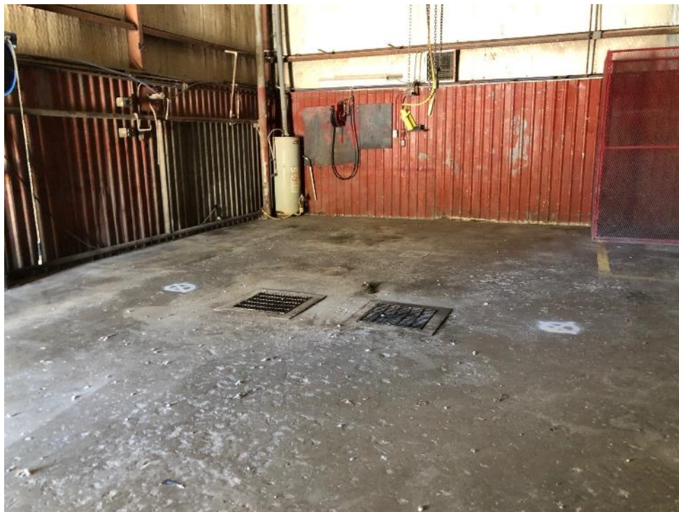
Photo 10 - Looking east at locations of DP-16 and DP-17 marked in white inside of Building 6
