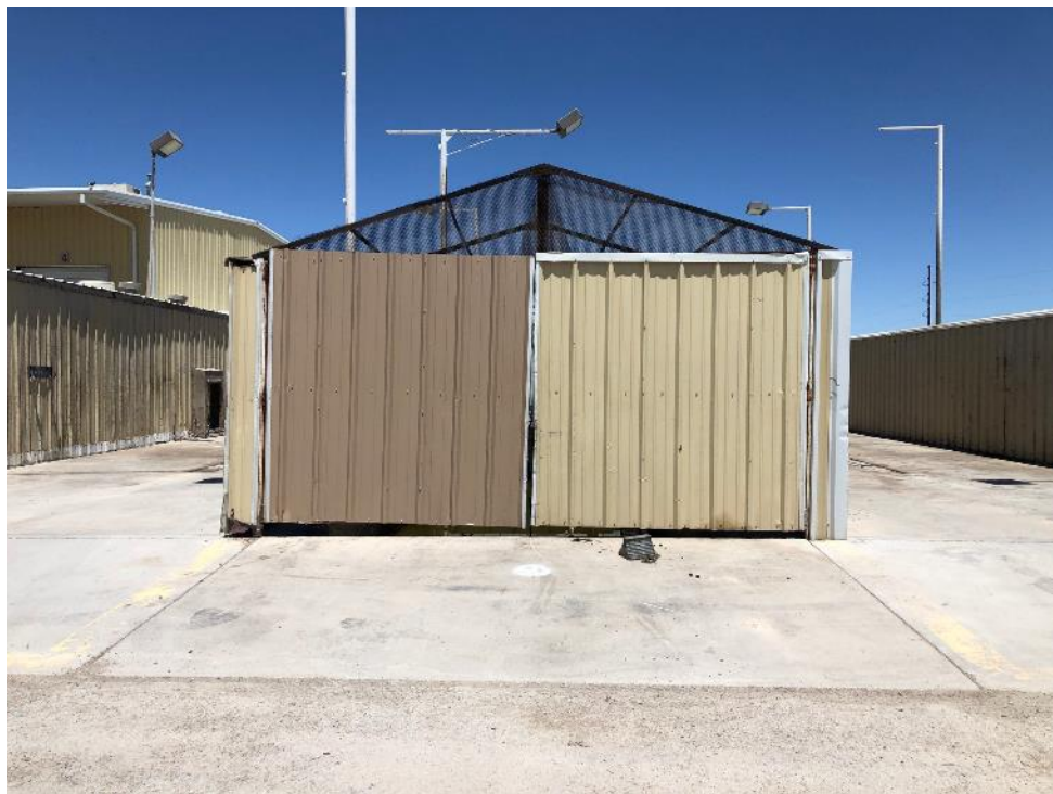
Photo 4 - Looking north at south side of the grit pit and DP-7 location marked in white
