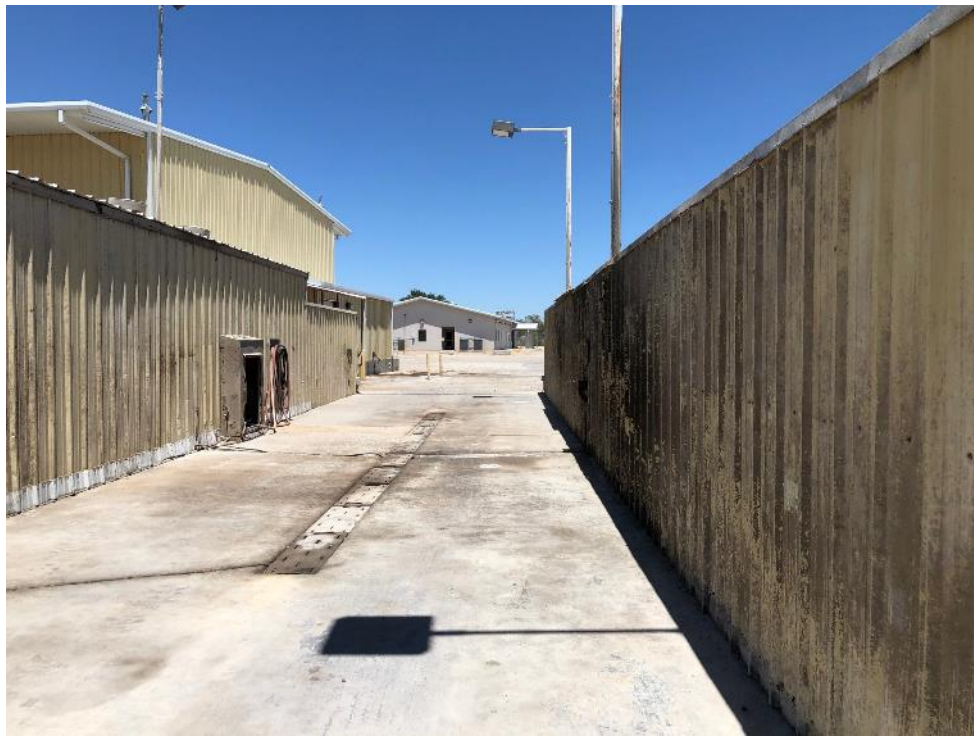
Photo 5 - Looking north through west wash bay at location of DP-8 in front of DP-9 marked in white
