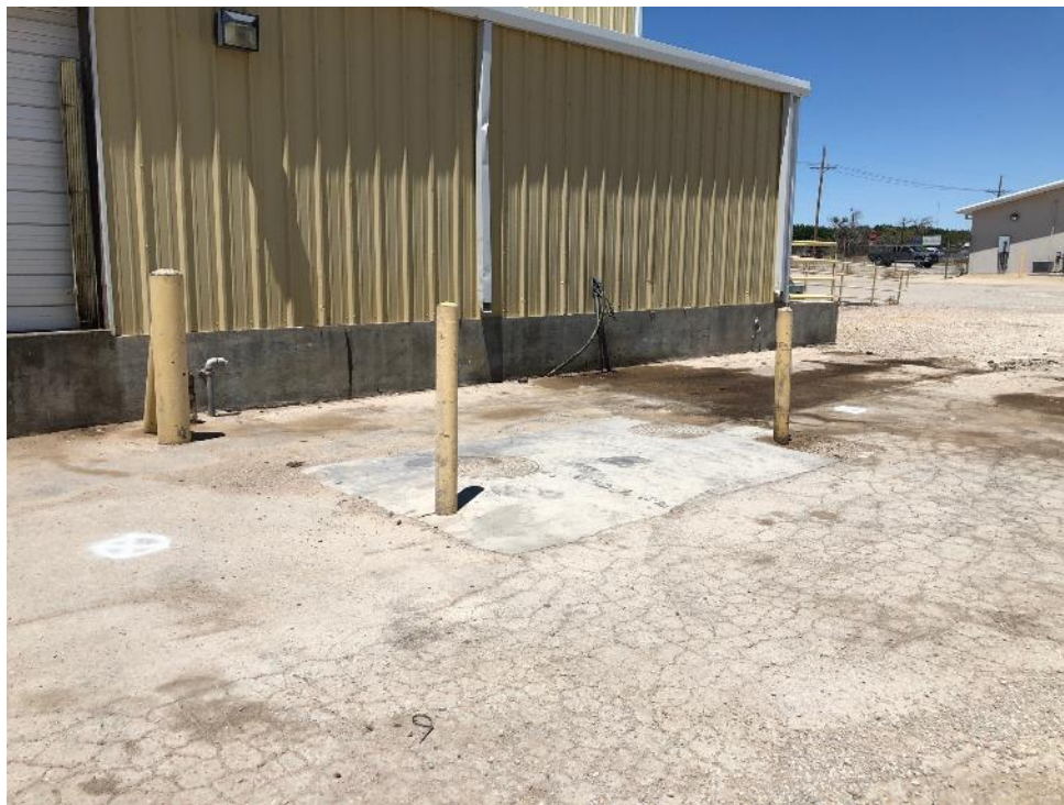
Photo 6 - Looking northwest at DP-10 and DP-11 marked in white on east side of building 3. Final location of both borings was shifted east to avoid underground piping.
