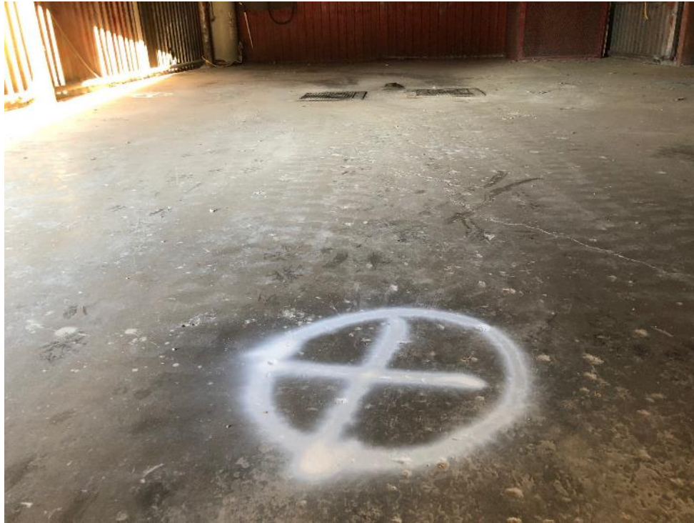
Photo 17 - Looking east at location of DP-24R marked in white inside of Building 6
