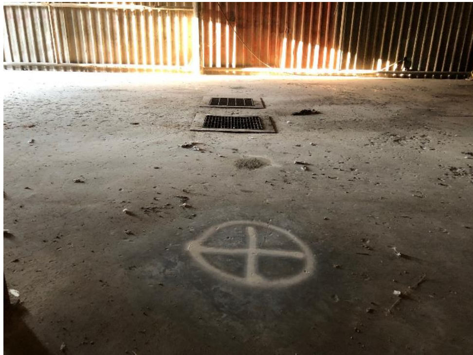
Photo 16 - Looking north at location of DP-23R marked in white inside of Building 6
