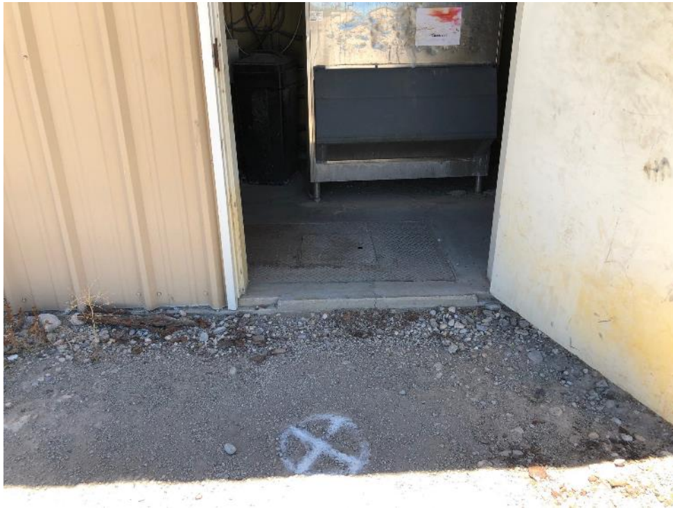
Photo 9 - Looking south at location of DP-15 marked in white near north end of Building 6
