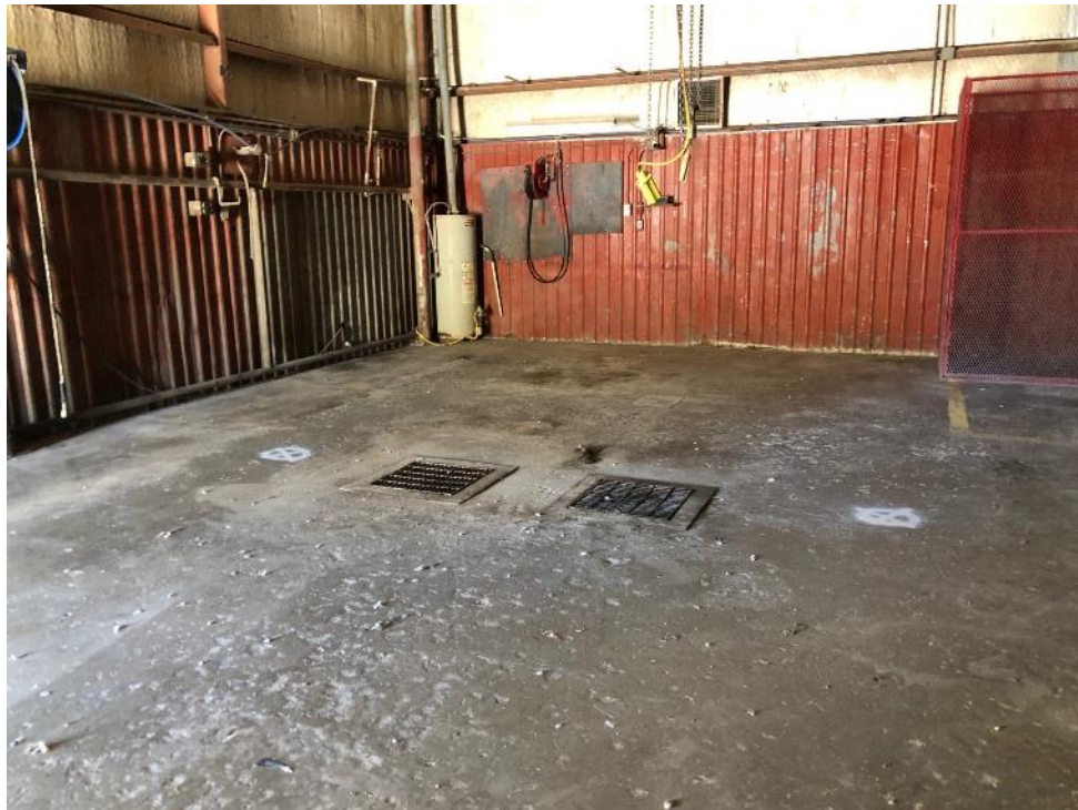
Photo 10 - Looking east at locations of DP-16 and DP-17 marked in white inside of Building 6
