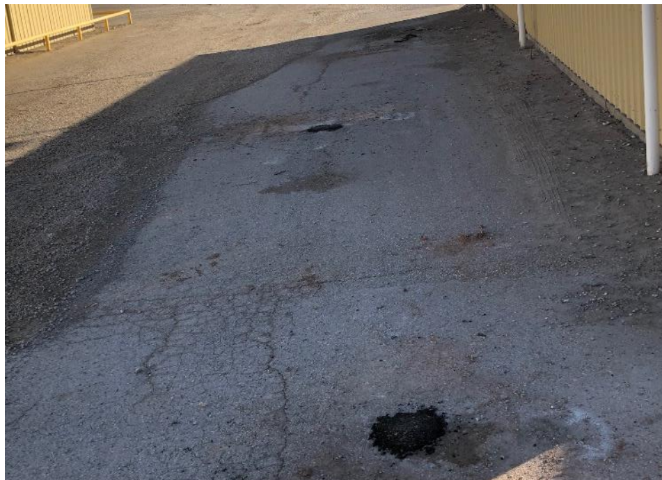
Photo 18 - Looking south at location of DP-25/25R and beyond at DP-26/26R marked by fresh black asphalt on east side of eastern wash bay
