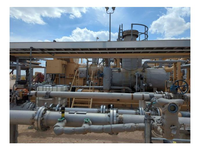
The lube oil DP was not functioning correctly. We had to shut down the compressor and pull strainer to fix DP issues. This was preventative maintenance in order to avoid a major shut event.
