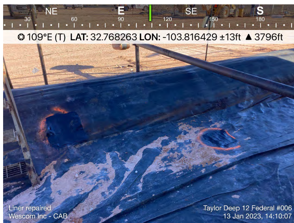
Liner holes repaired
