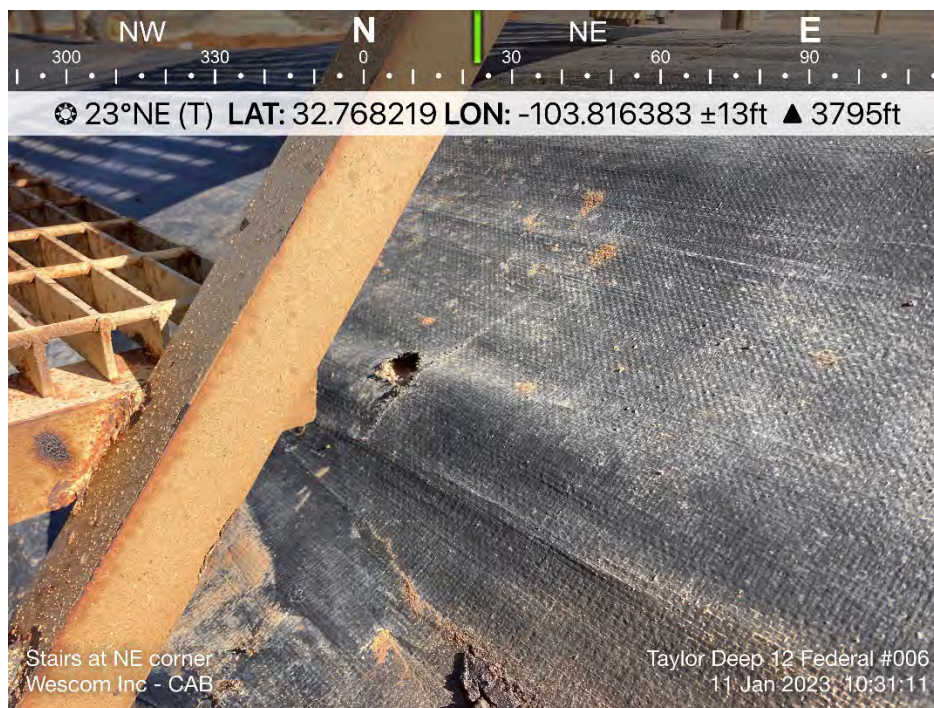
Hole in liner behind stairs (SS12)
