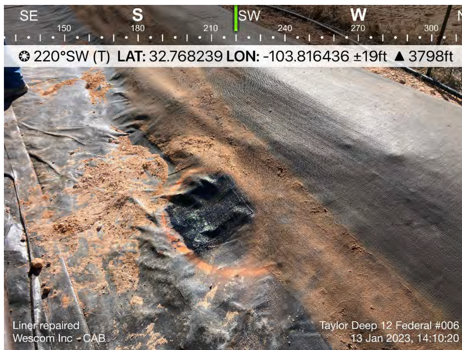
Liner holes repaired
