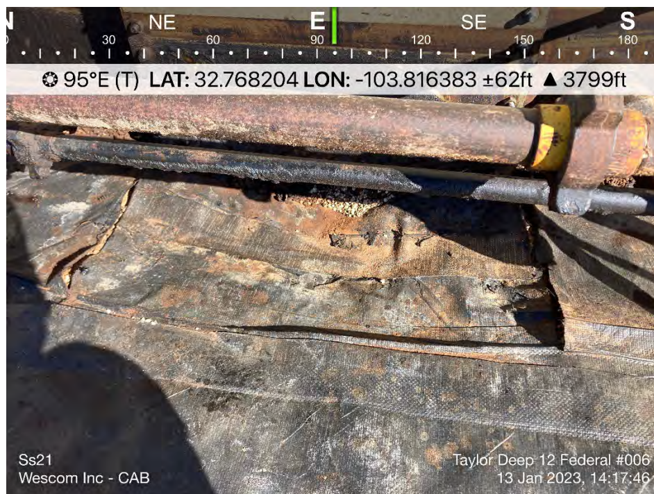
Liner separation behind center tank and delineation under liner (SS21)
