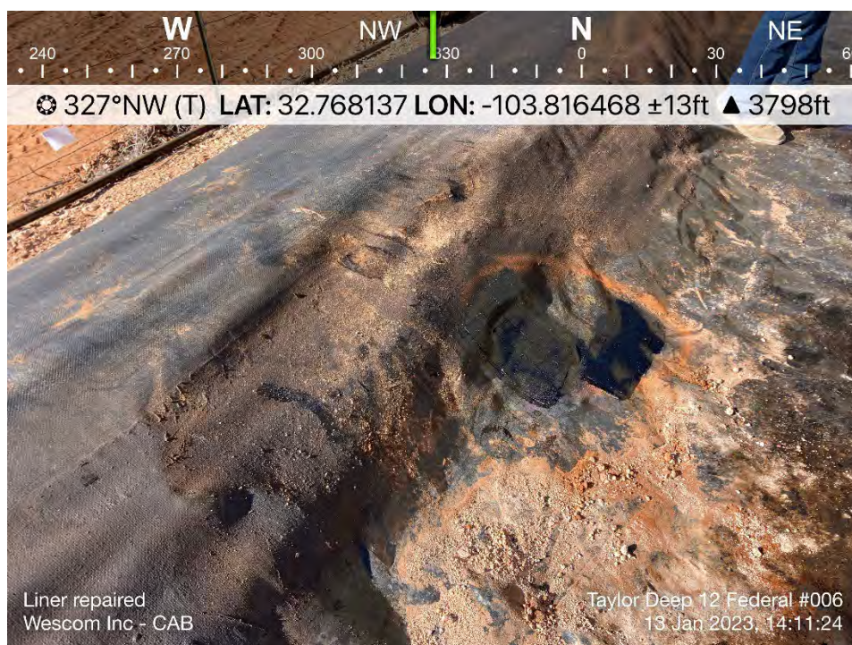
Liner holes repaired
