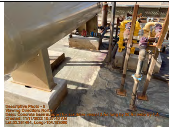
Three Concrete base support for scrubber vessel and yellow pneumatic pump. 3' long by 20" wide by 1' tall
