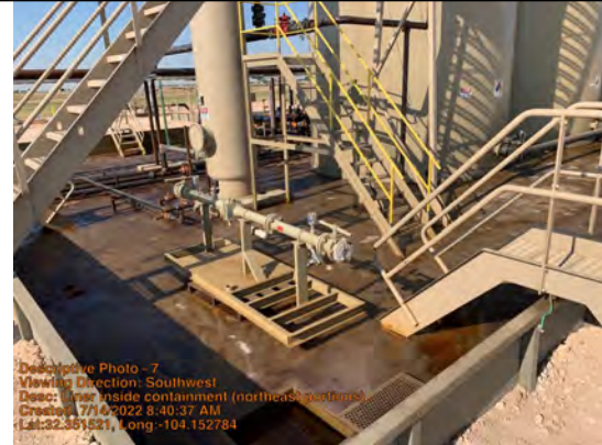
Liner inside containment (northeast portions)
