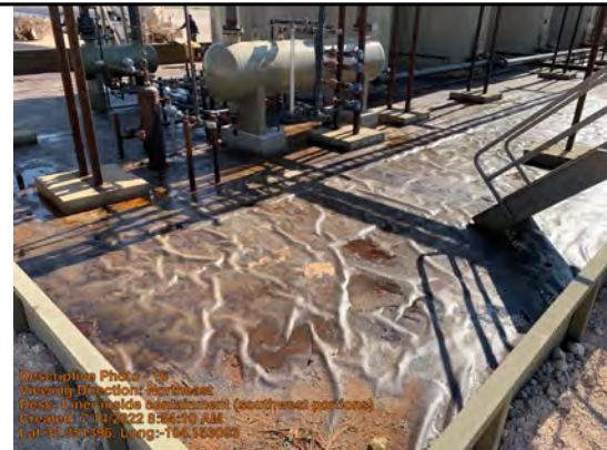
Liner inside containment (southwest portions)
