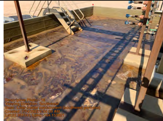
Liner inside containment (southwest portions)
