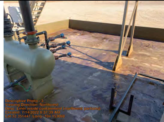
Liner inside containment (northwest portions)
