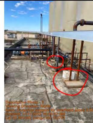
10 Concrete support bases within containment for overhead pipes 3' wide by 3' long by 6" tall
