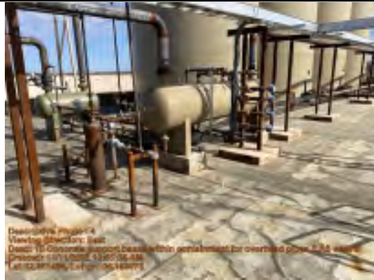
Concrete support bases within containment
