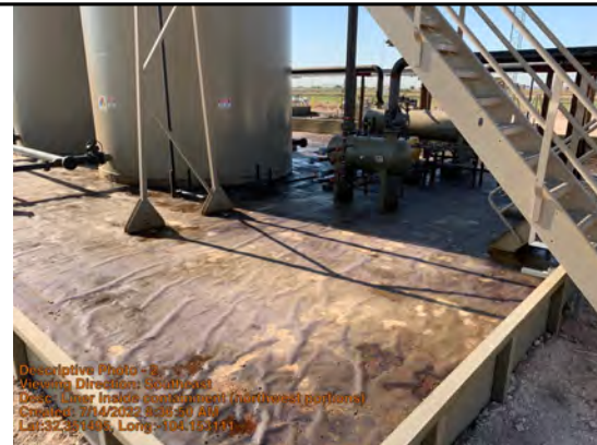
Liner inside containment (northwest portions)
