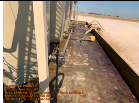
Liner inside containment (northern portions)
