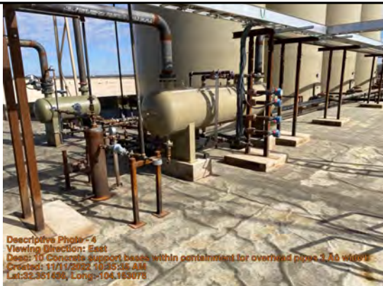
10 Concrete support bases within containment for overhead pipes 3' wide by 3' long by 6" tall
