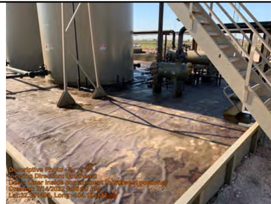
Liner inside containment (northwest portions)
