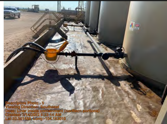
Liner inside containment (northern portions)
