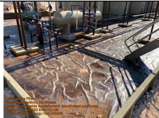
Liner inside containment (southwest portions)
