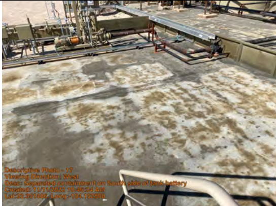
Separated containment on South side of tank battery
