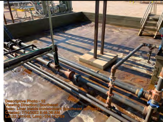
Liner inside containment (southeast portions)
