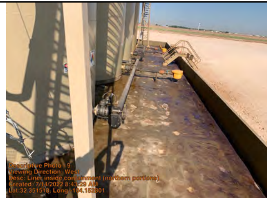
Liner inside containment (northern portions)
