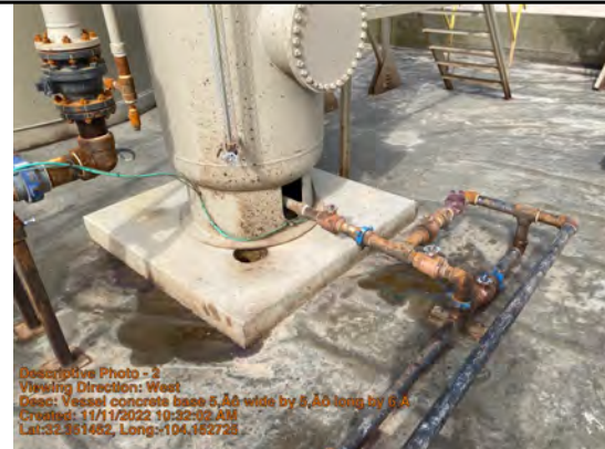
Vessel concrete base 5' wide by 5' long by 6" tall
