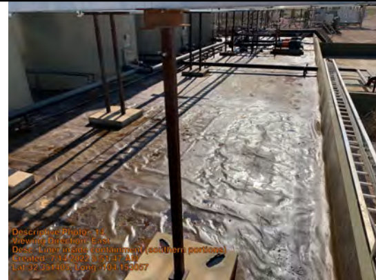
Liner inside containment (southern portions)
