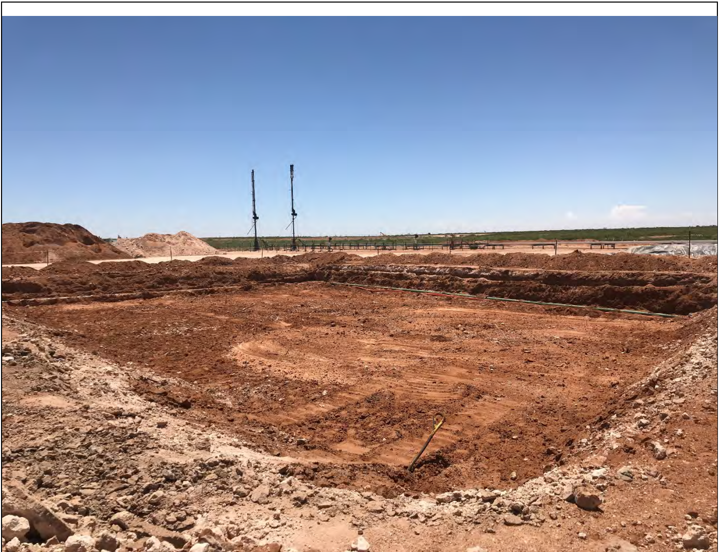
Southeast facing view of the southern portion of the excavation.
