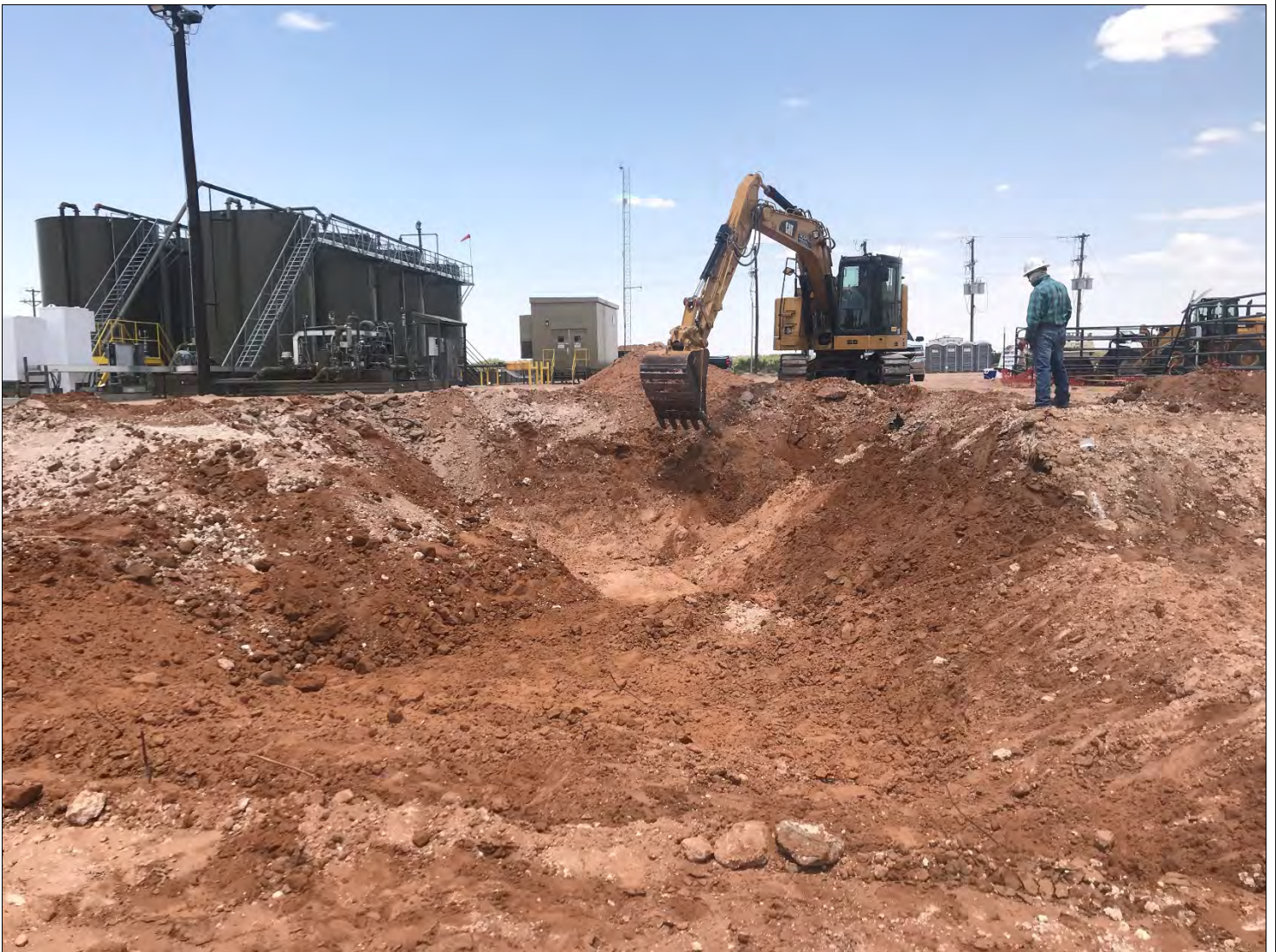
North facing view of the central portion of the excavation.
