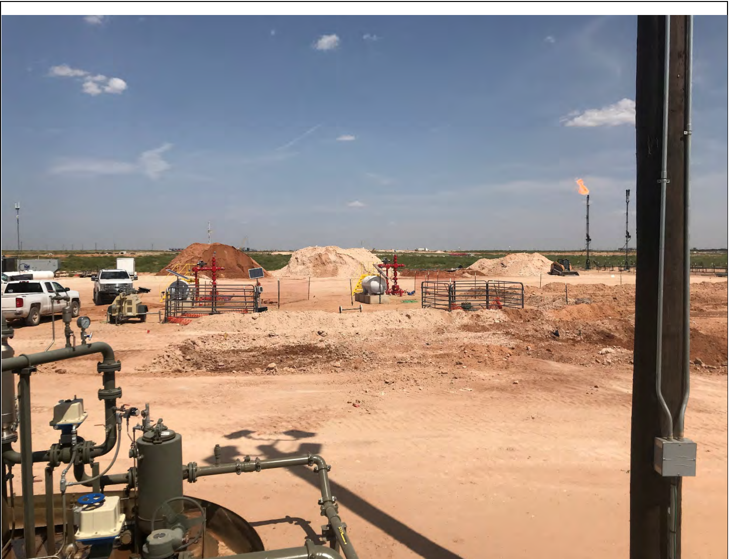
East facing view of the northern portion of the excavation.
