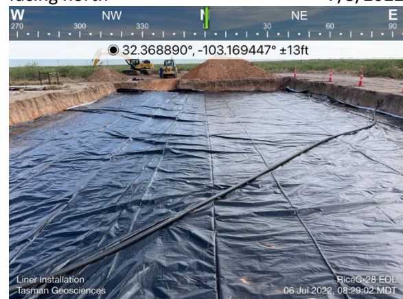
20-mil reinforced liner installed at 4.5 ft bgs, facing north
