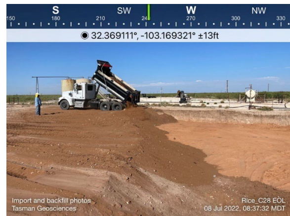
Backfilling above the 20-mil liner previously padded with imported blow sand
