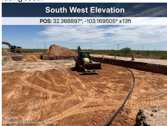
Padding the excavation with imported blow sand, facing north
