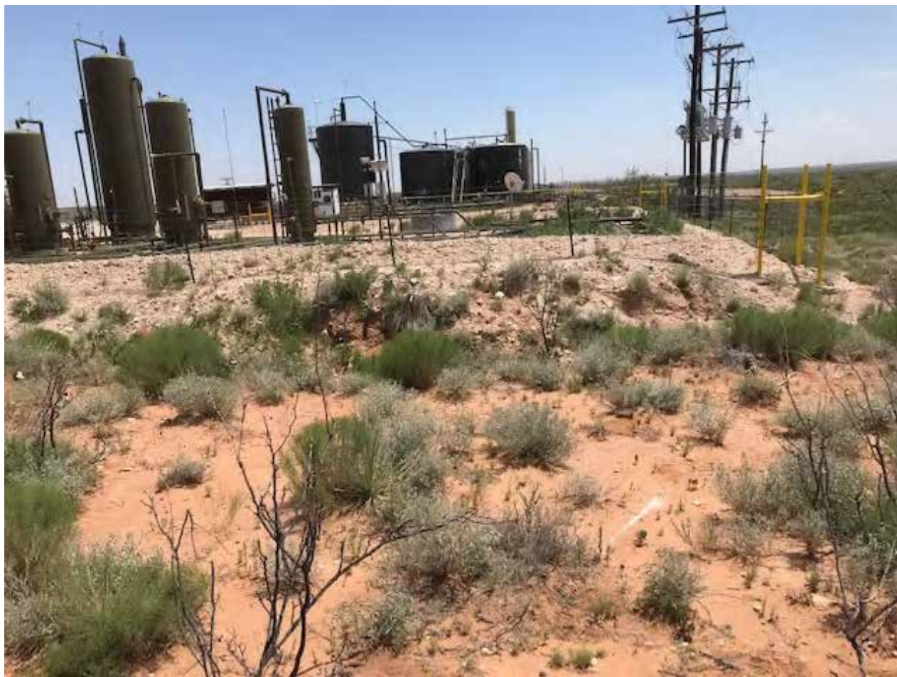
South facing view of release/assessment area (2RP-4396, 2RP-4397).
