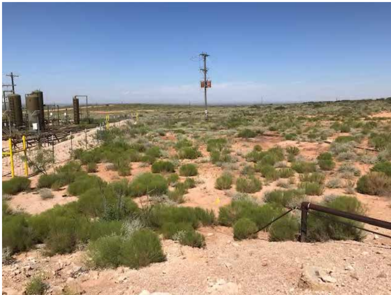
West facing view of pasture area north of the process equipment (2RP-4396, 2RP-4397).
