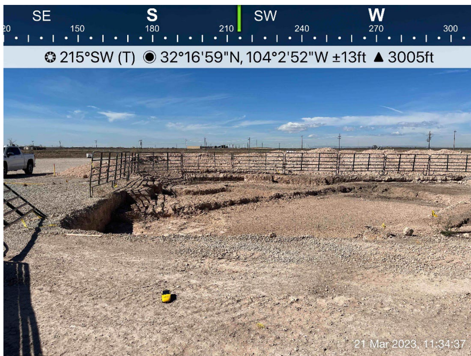
Excavated area viewing southwest, March 21, 2023
