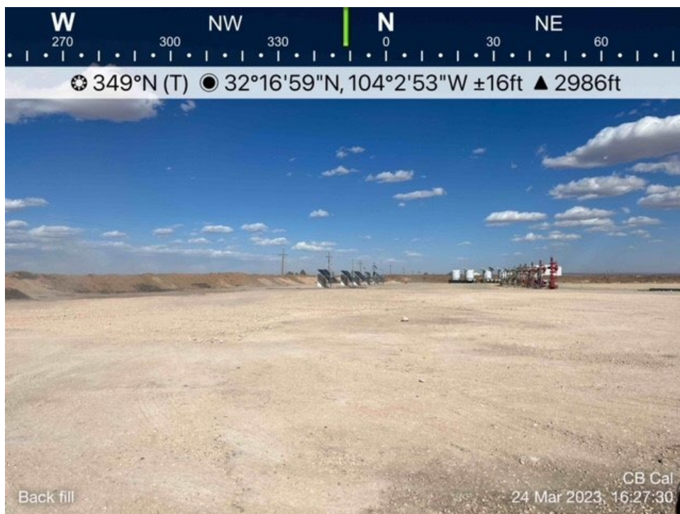
Backfilled excavation viewing north, March 24, 2023
