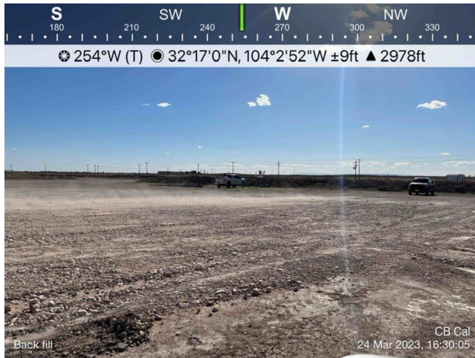
Backfilled excavation viewing west, March 24, 2023
