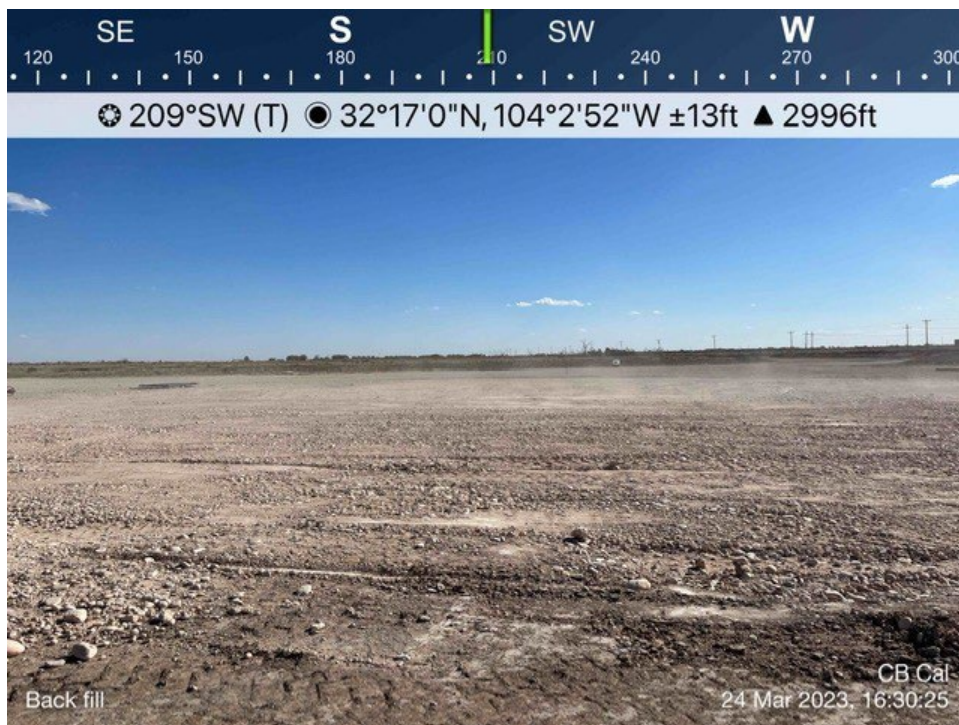
Backfilled excavation viewing southwest, March 21, 2023
