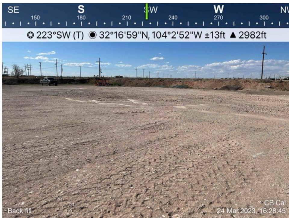
Backfilled excavation viewing southwest, March 24, 2023
