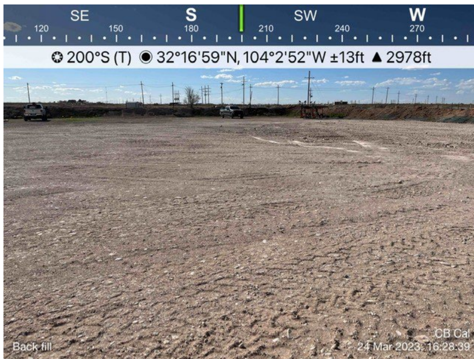
Backfilled excavation viewing south, March 24, 2023
