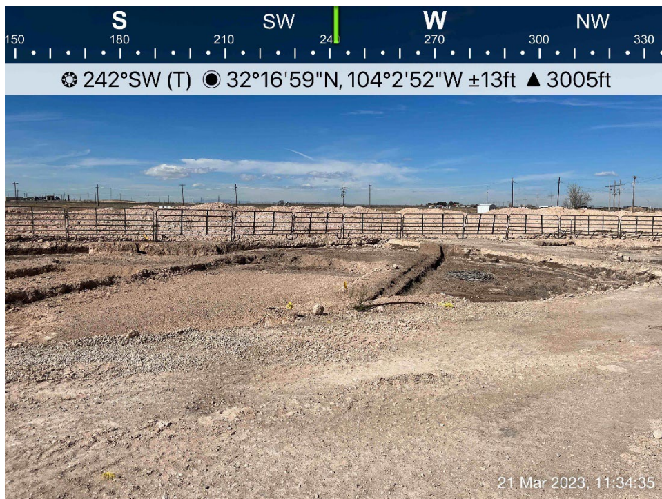
Excavated area viewing southwest, March 21, 2023
