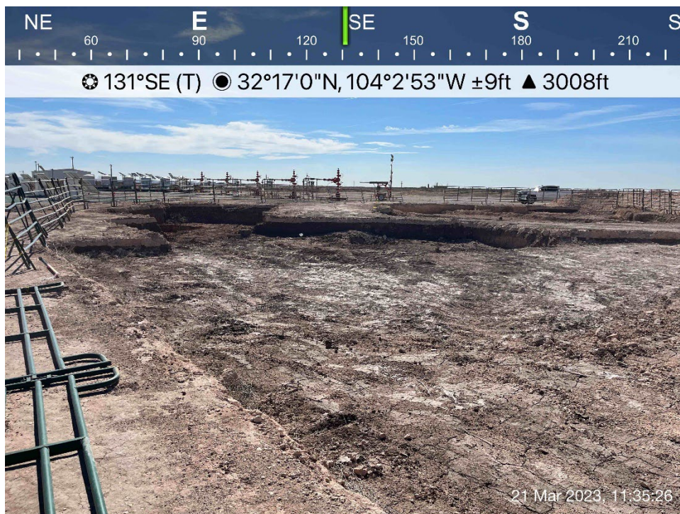
Excavated area viewing southeast, March 21, 2023
