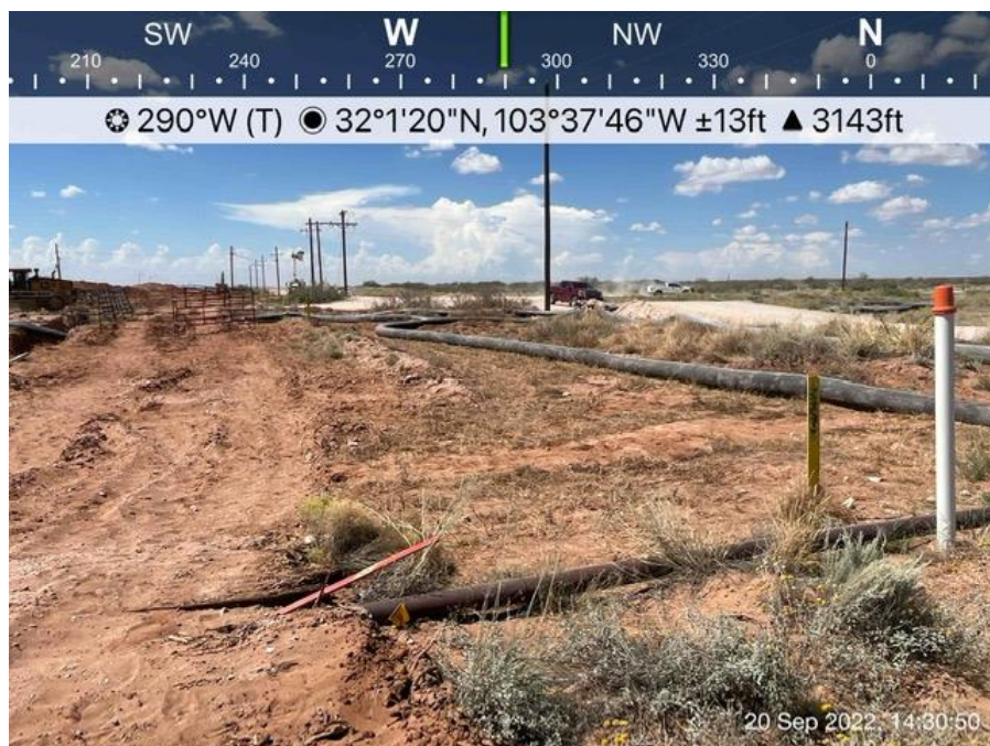
Impacted Area view from the west-northwest September, 20, 2022.
