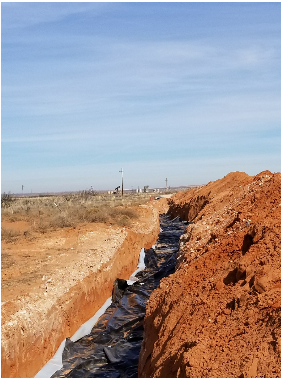
Photo 1 - Liner Placement
