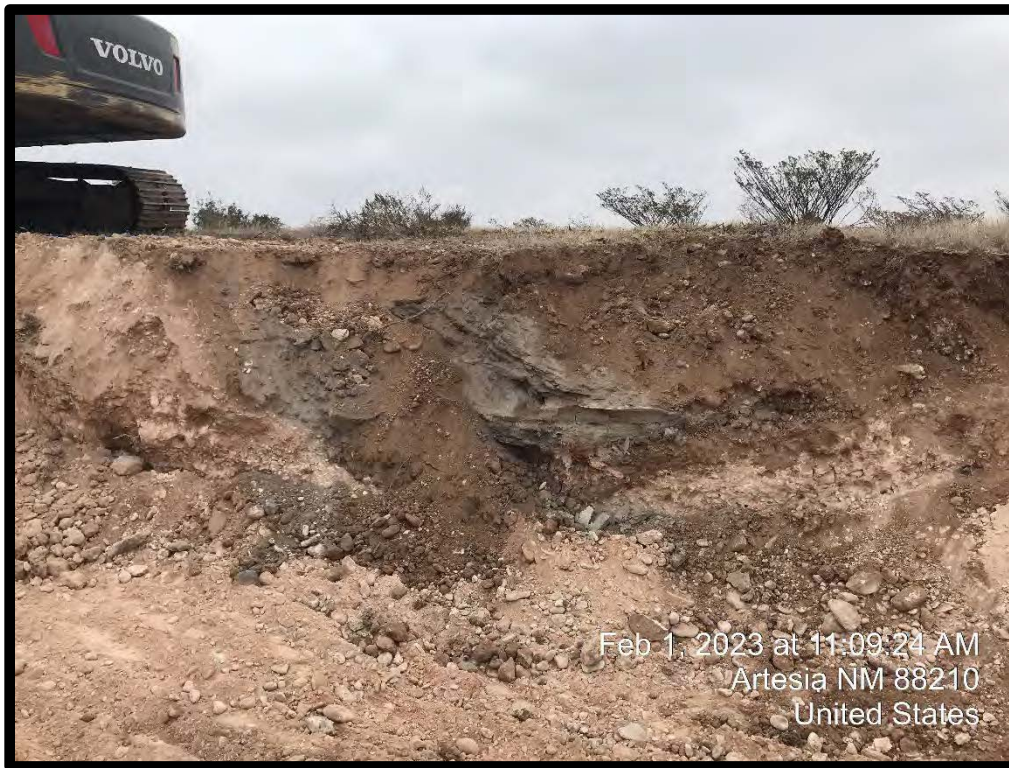
PHOTOGRAPH NO. 5 – A view of historic pit material encountered in the northern wall of the “Northeastern Excavation Area”. The view is towards the north-northwest.
